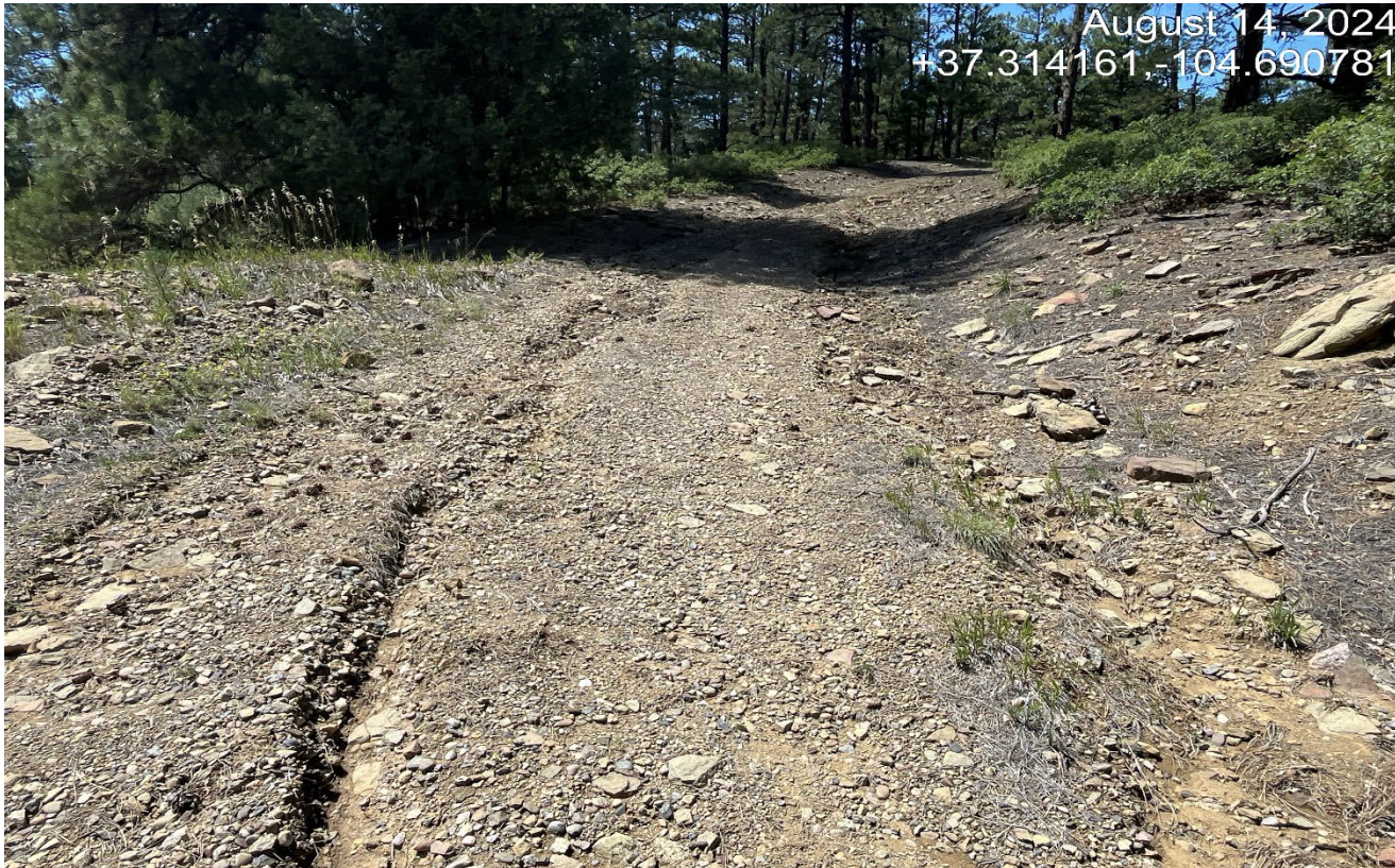
Photo 1. Facing northwest toward the access road. There is erosion along the road that will need to be repaired.
