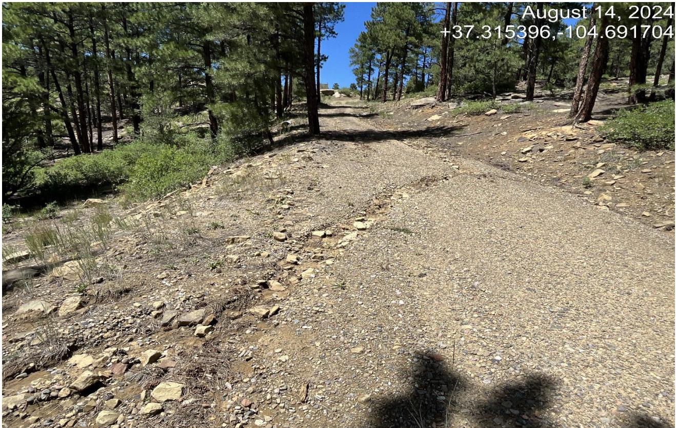
Photo 2. Facing northwest along the access road. Stormwater is bypassing the culvert and is causing erosion of the road.
