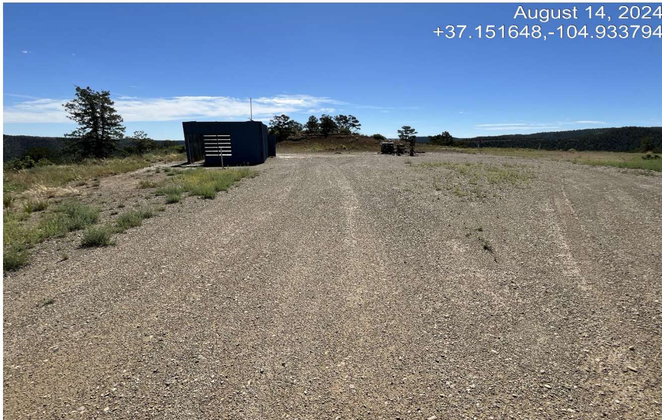
Photo 1. Facing east toward the wellsite.
