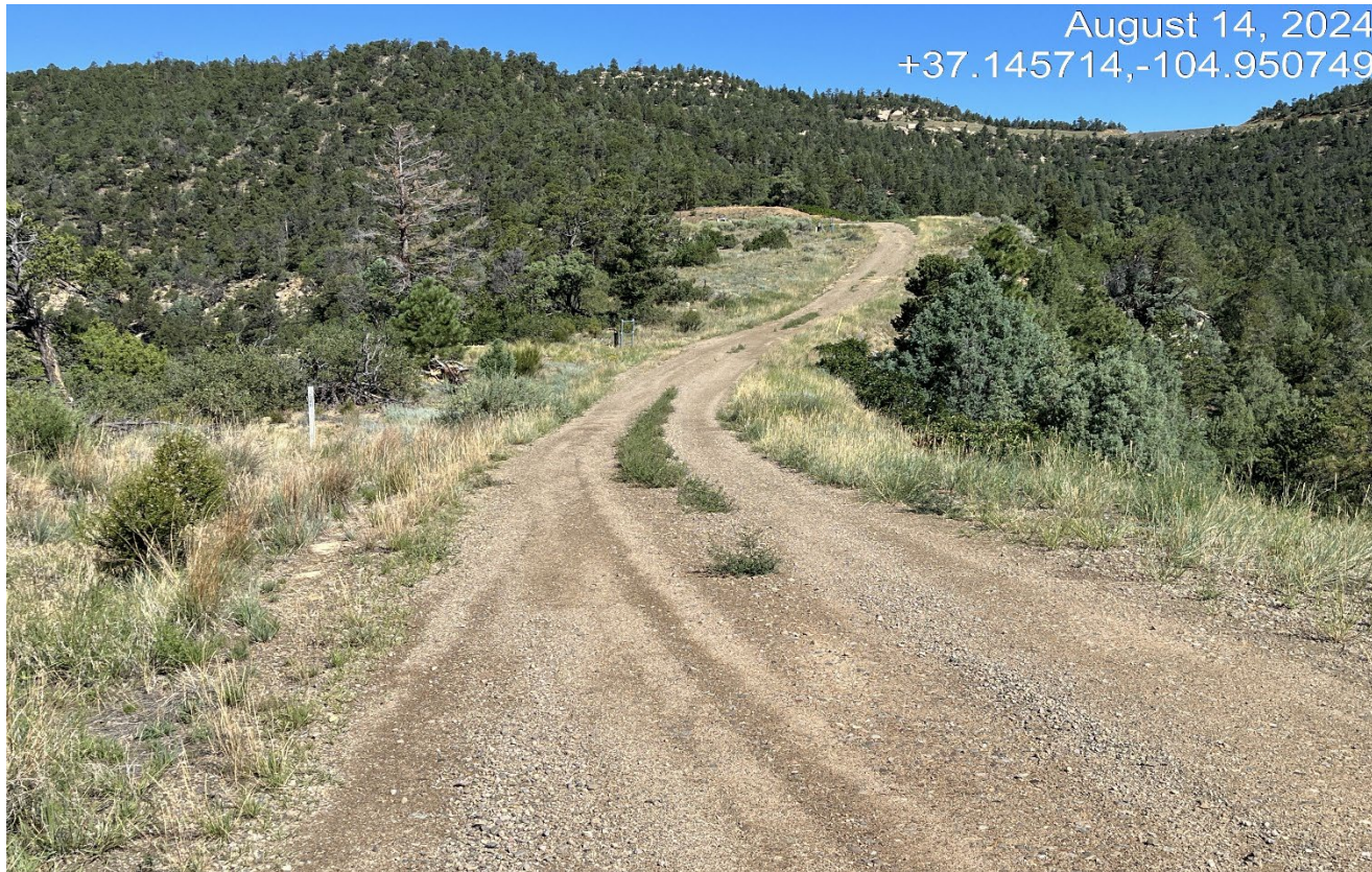
Photo 2. Facing northwest along the access road.
