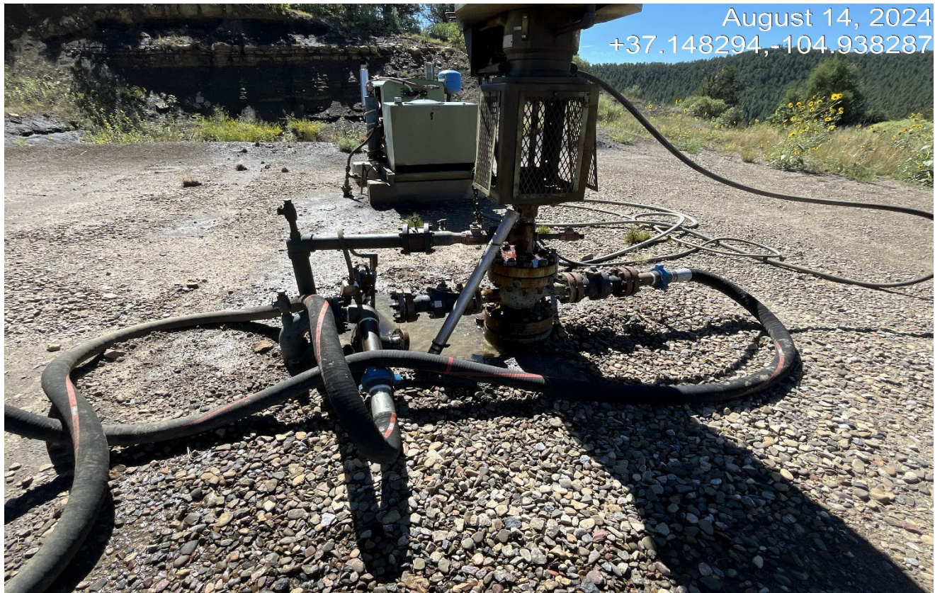
Photo 3. There is water dribbling out of the wellhead that needs to be fixed..
