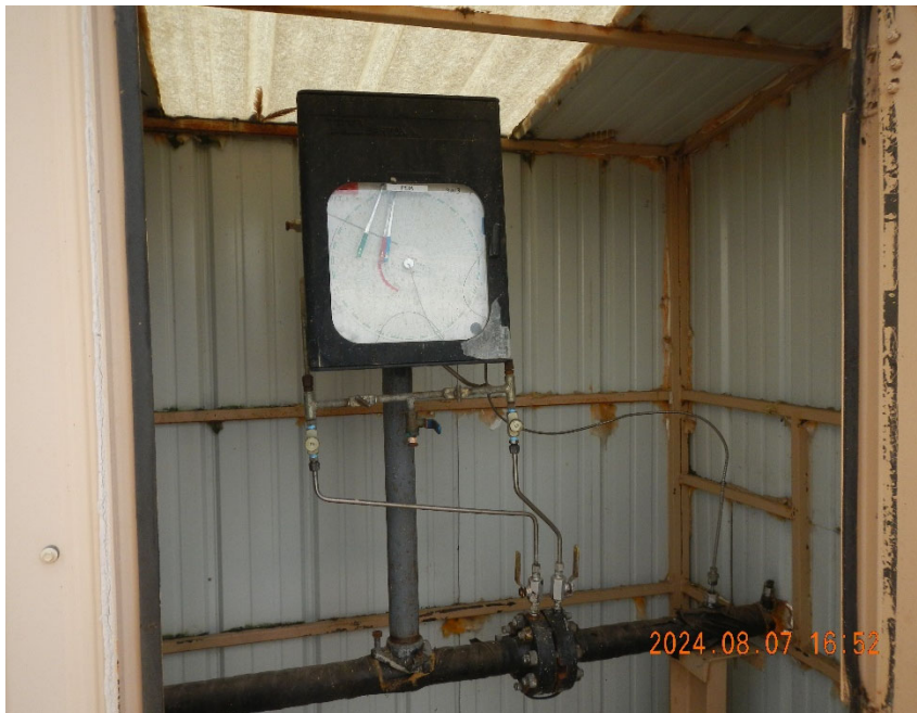
3. Gas meter inside meter shed.
