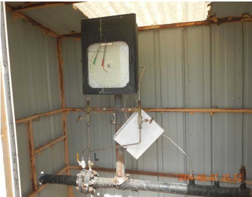
3. Gas meter inside meter shed.
