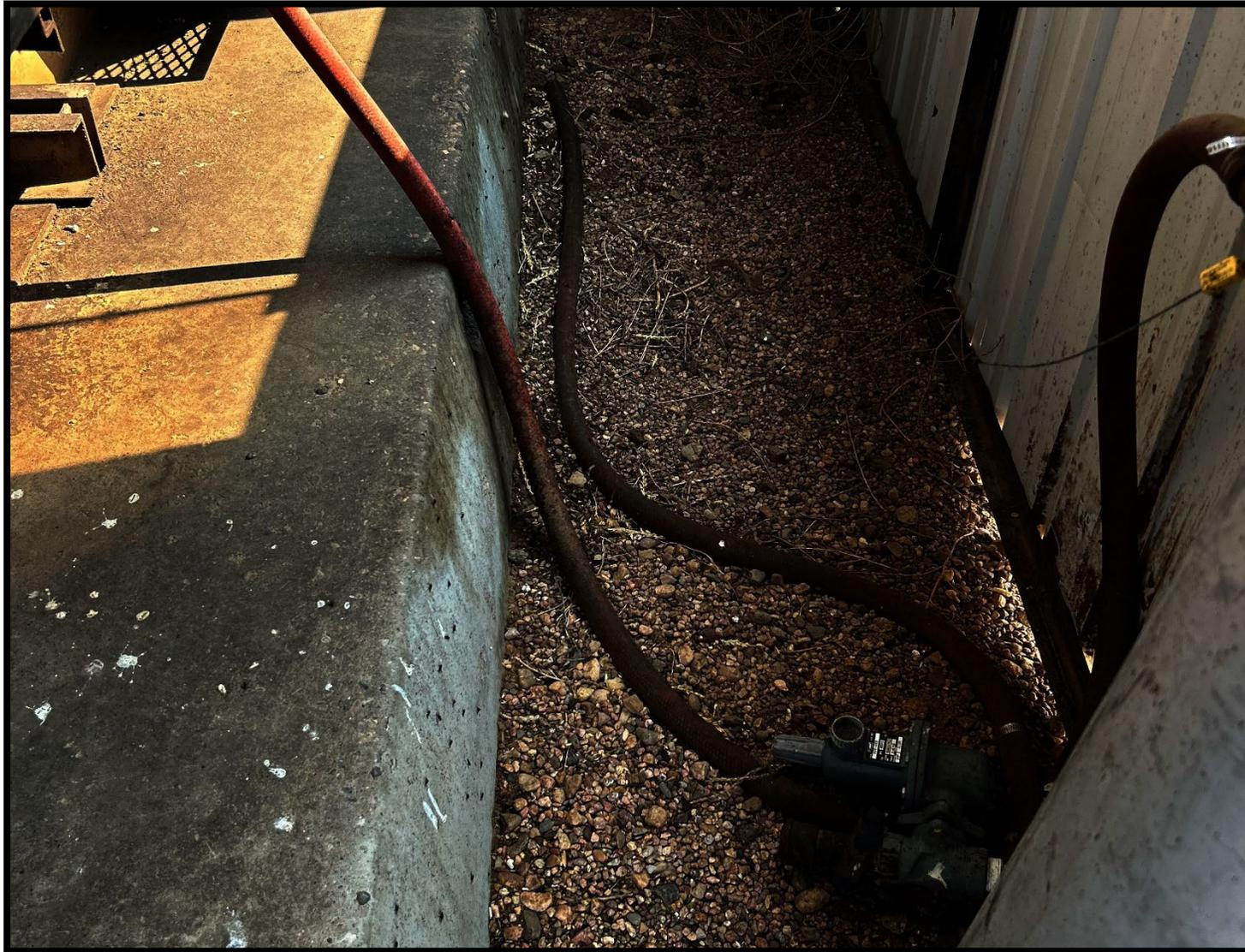
**CA:** Stained Soil at Exhaust and Gas Engine, see photos 3, 4, & 5. Mechanical condition Comply with Rule 605.d. Properly treat or dispose of oily waste in accordance with 907.e.
