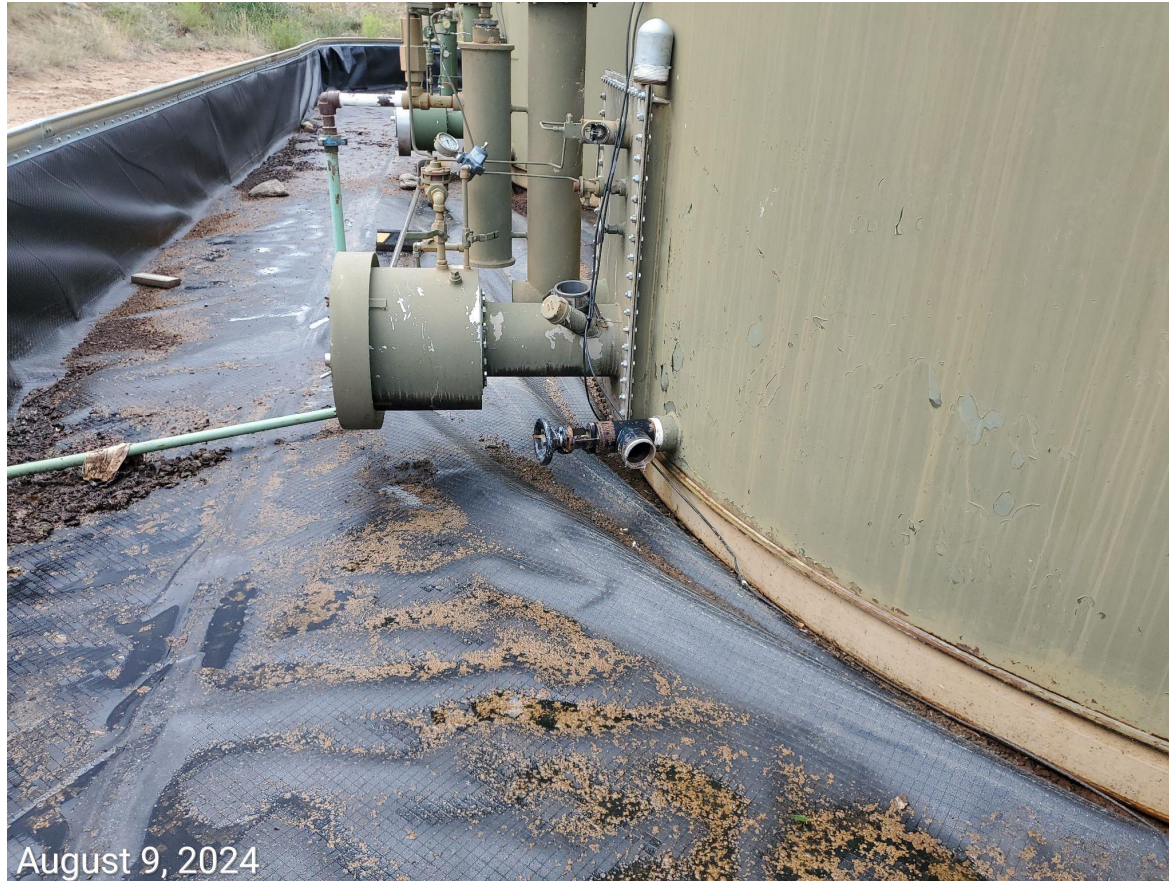
Photo 4: Cap/Plug remain missing from lines at tank.
