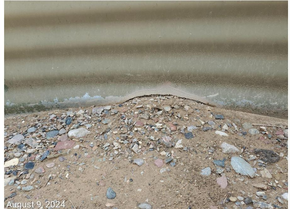
**Photo 5:** Photos 5-6 taken from the battery facility. Photo shows holes within the metal containment berm. Work to ensure BMP remains sufficiently impervious to contain a spill or release have not been taken.
