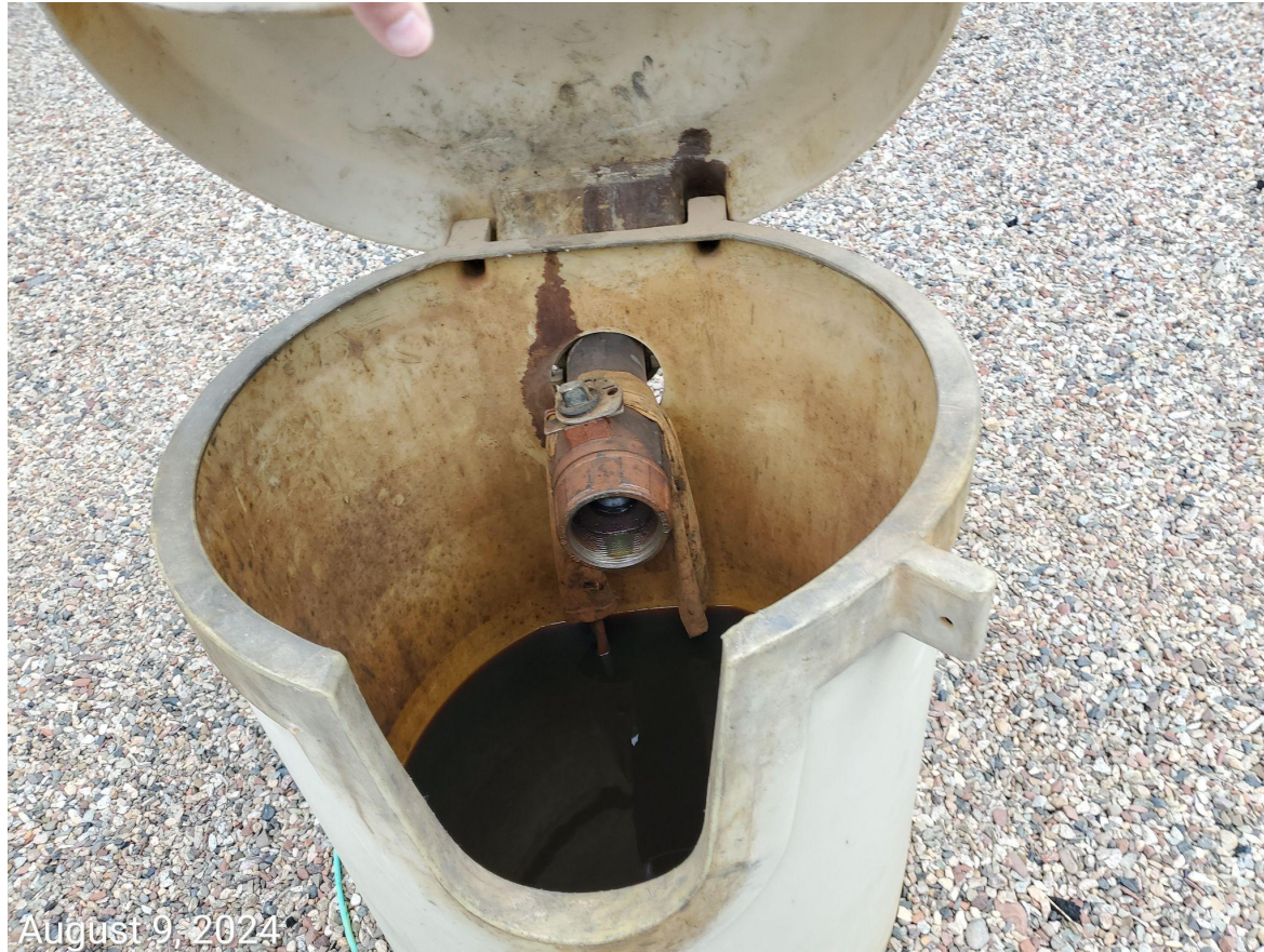
Photo 3: Lines at tank missing cap/plug. Produced fluids within containment.
