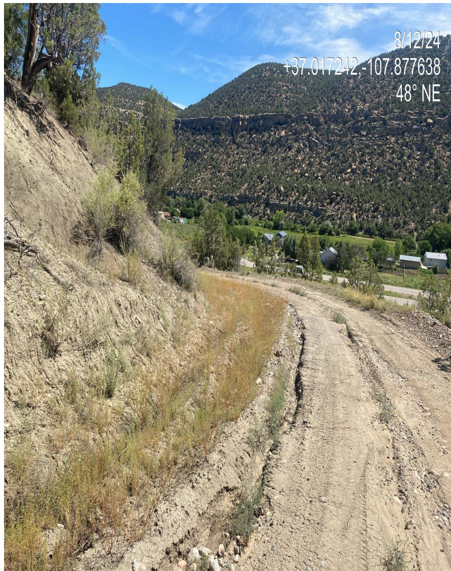
Photo 3. View of stormwater issues observed along the access road. Additional stabilization is needed to minimize degradation to the access road.
