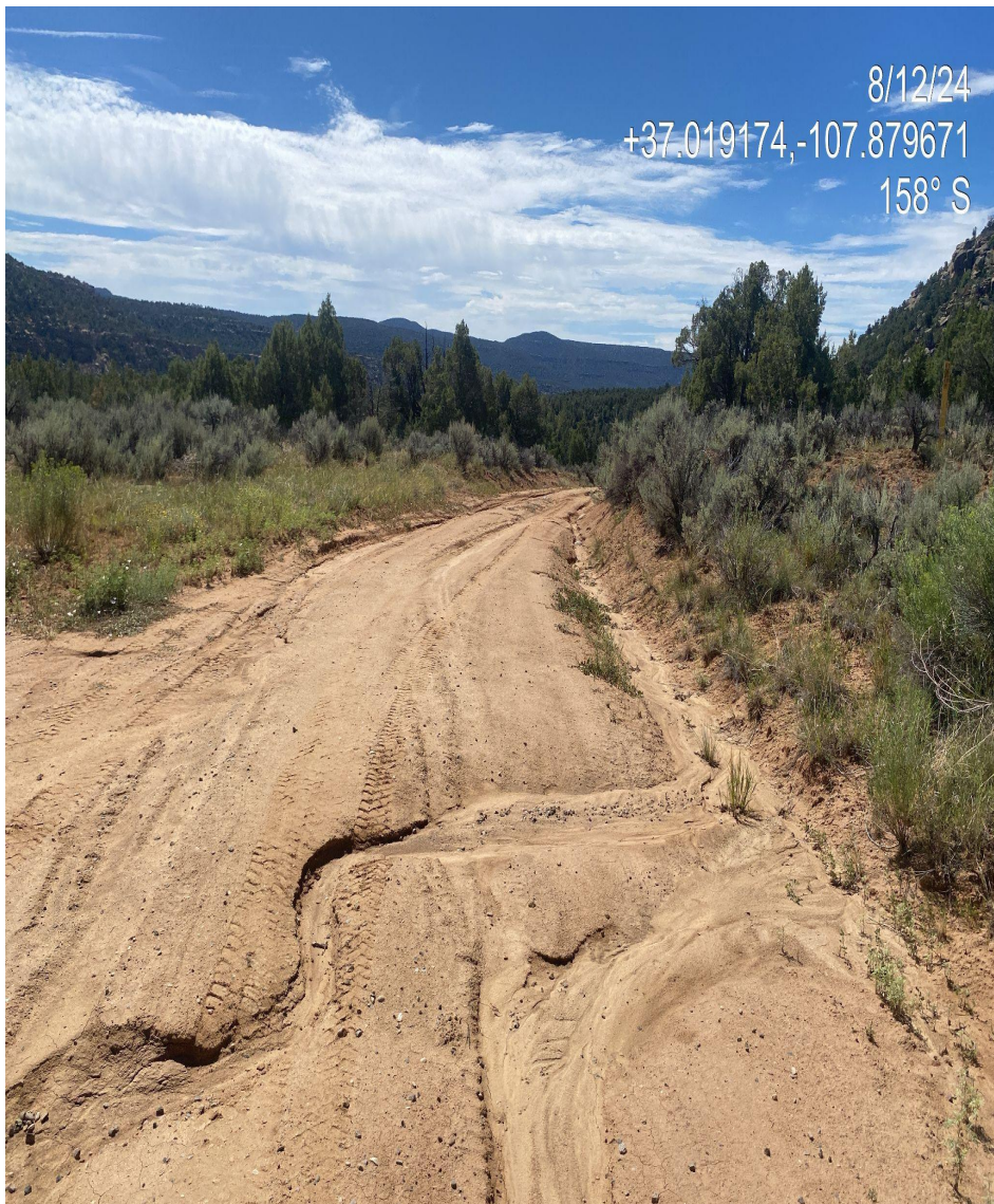
Photo 3. View of stormwater issues observed along the access road. Additional stabilization is needed to minimize degradation to the access road.
