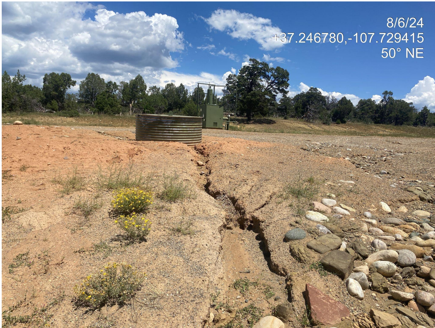
Photo 3. View of rill/gully erosion forming in the southwest corner of the disturbance. Storm water BMPs/controls are needed in this area.
