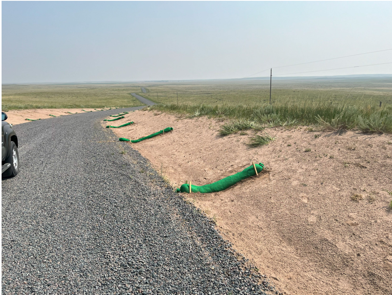
Photo 4: Erosion repair along the road to the well pad (Photo July 25, 2024).
