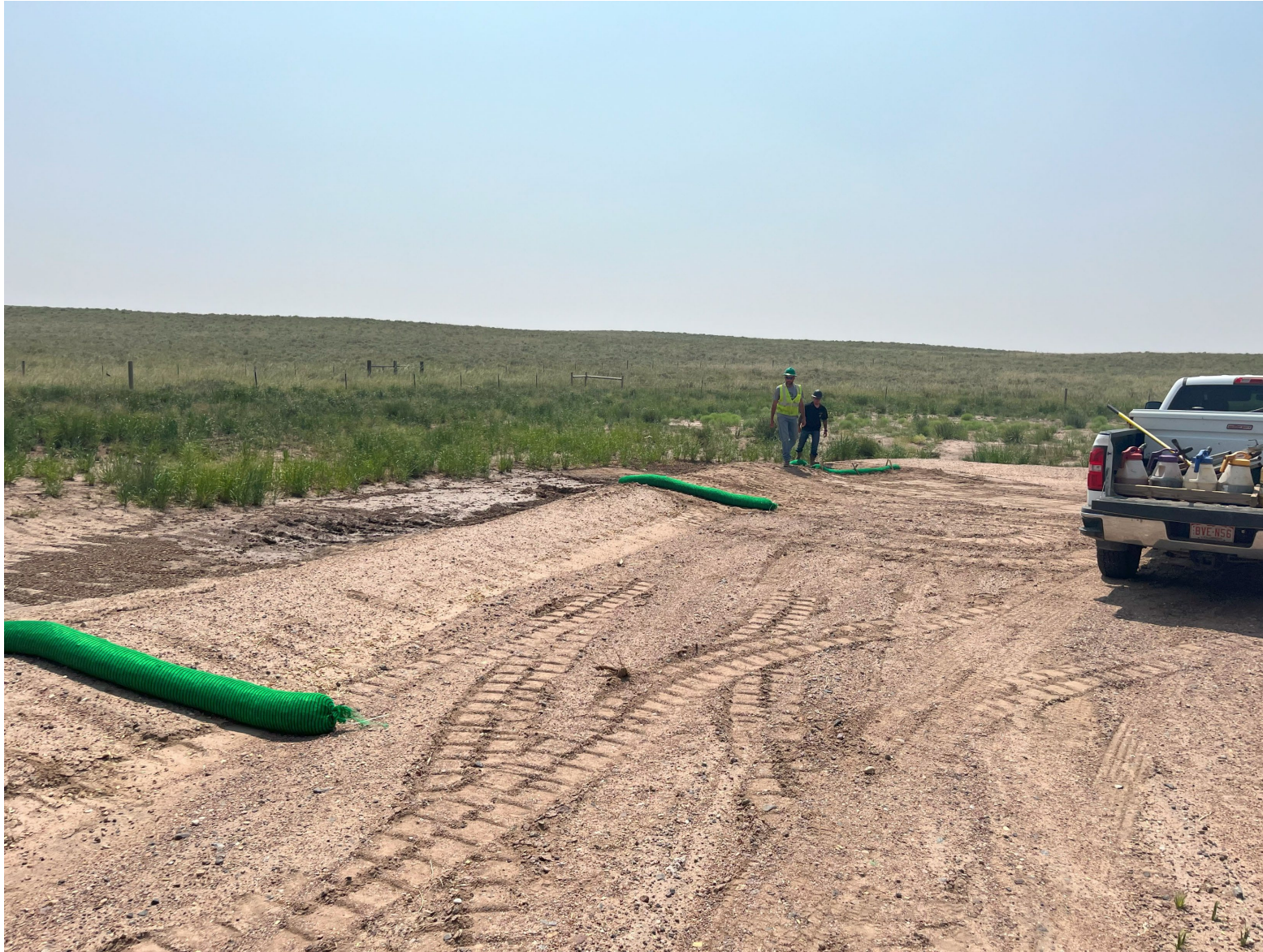
Photo 8: Erosion repair and BMP installation on the well pad (Photo July 25, 2024).
