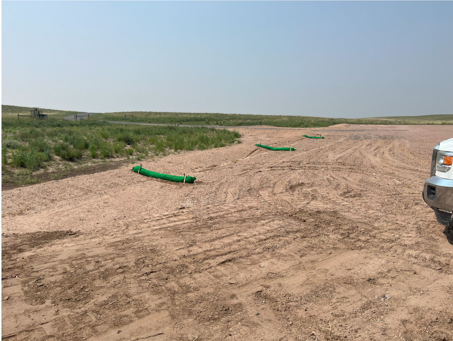
Photo 10: Erosion repair and BMP installation on the well pad (Photo July 25, 2024).
