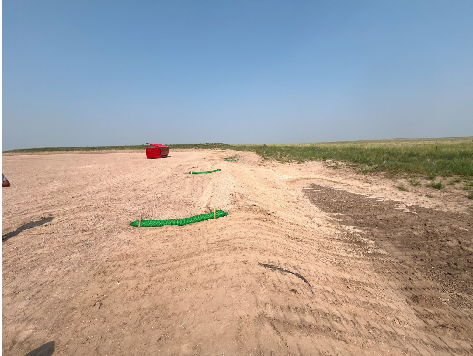
Photo 12: Erosion repair and BMP installation on the well pad (Photo July 25, 2024).
