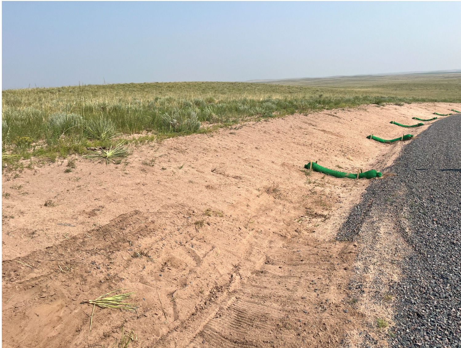
Photo 3: Erosion repair along the road to the well pad (Photo July 25, 2024).
