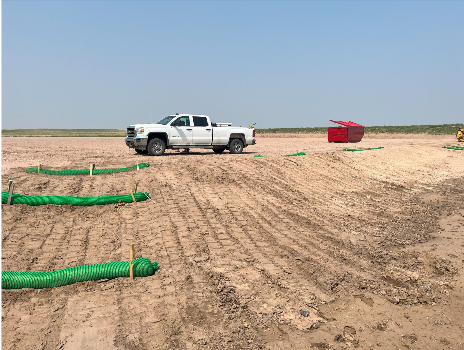
Photo 9: Erosion repair and BMP installation on the well pad
