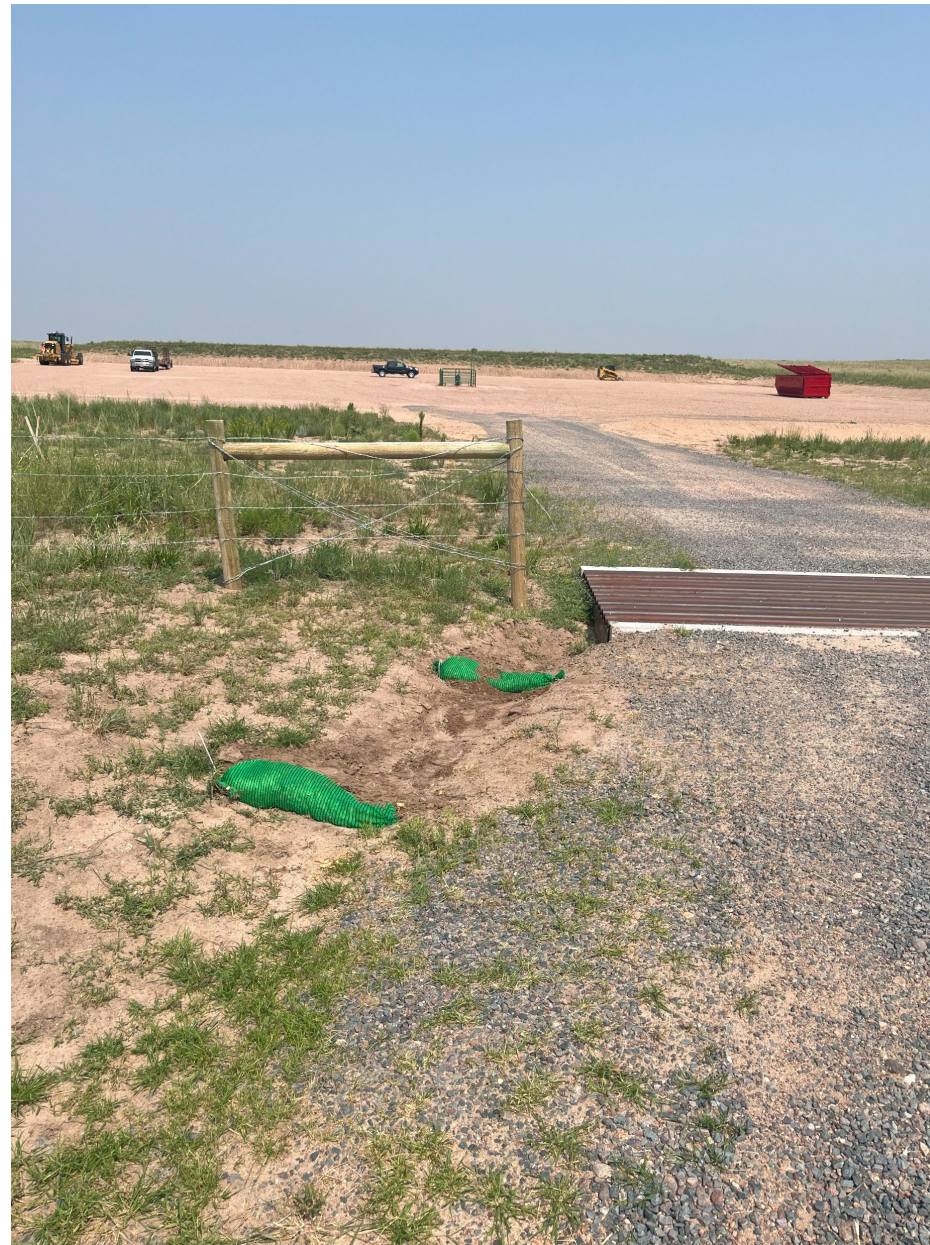
Photo 2: Erosion repair near the cattle guard and entrance to the well pad (Photo July 25, 2024).
