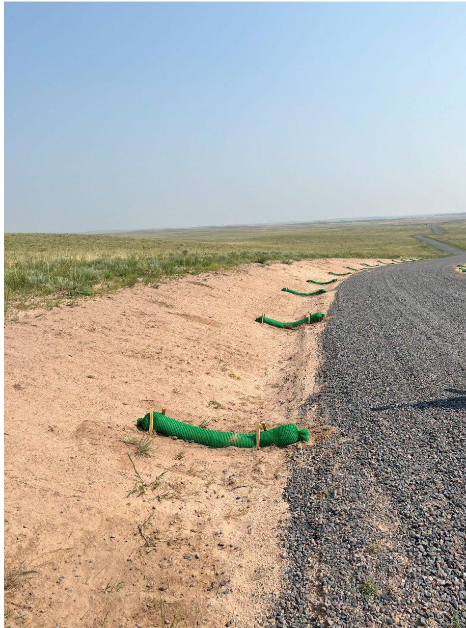
Photo 5: Erosion repair along the road to the well pad (Photo July 25, 2024).
