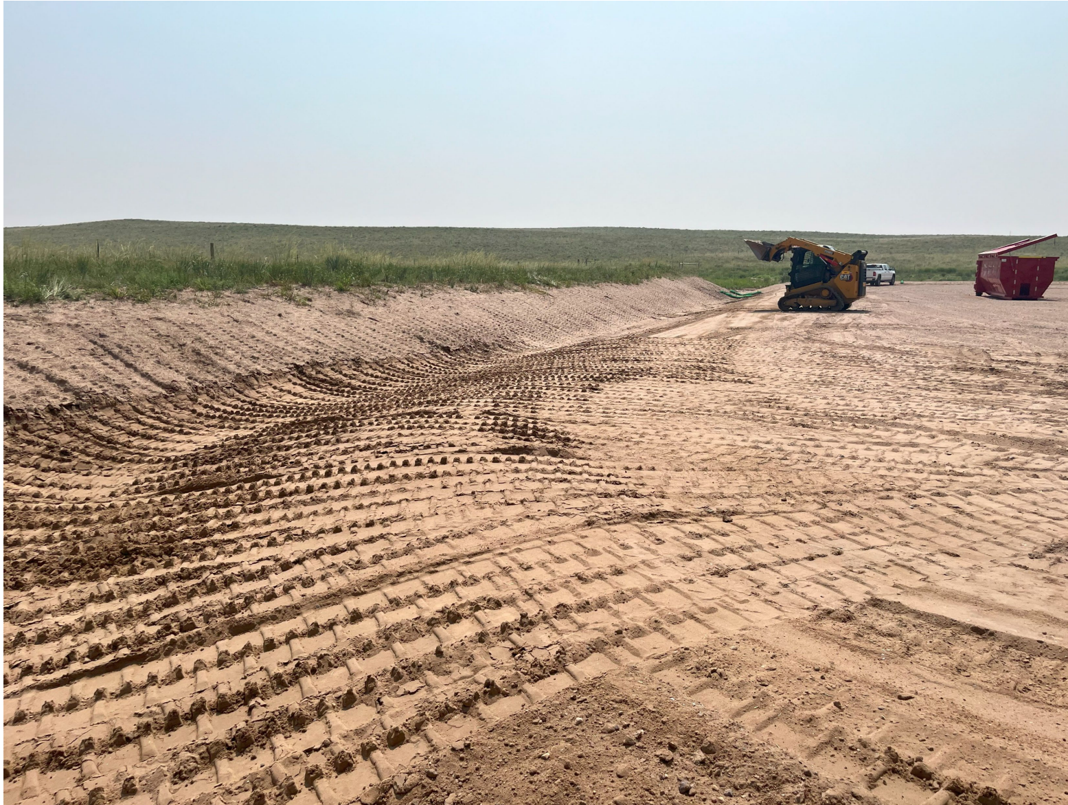
Photo 11: Erosion repair and BMP installation on the well pad (Photo July 25, 2024).
