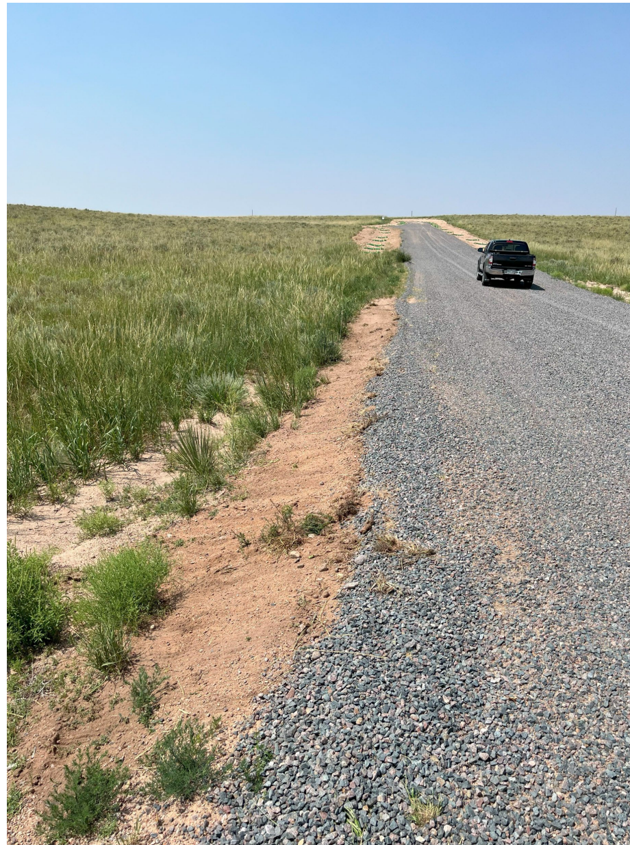
Photo 7: Erosion repair along the road to the well pad (Photo July 25, 2024).
