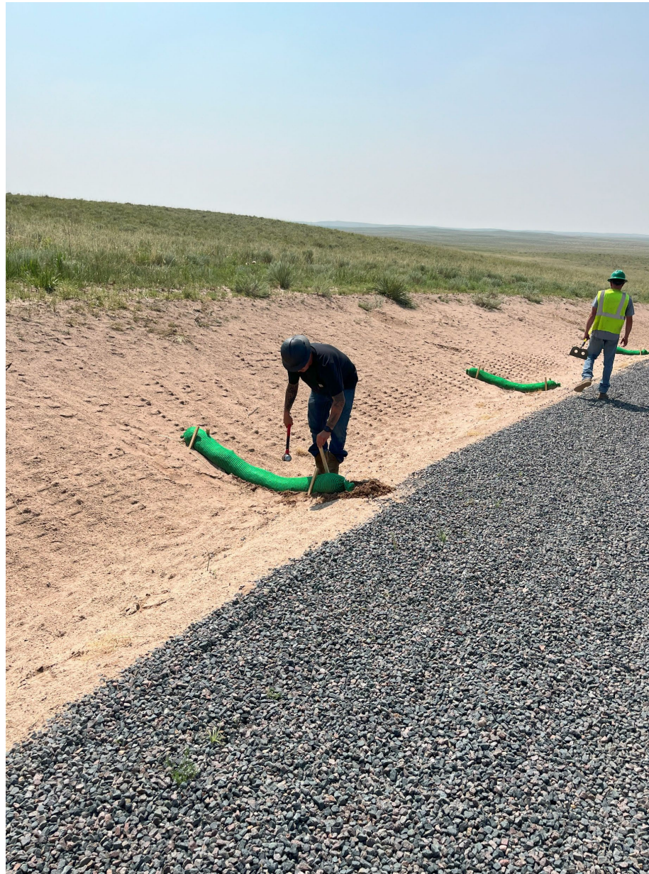
Photo 6: Erosion repair along the road to the well pad (Photo July 25, 2024).
