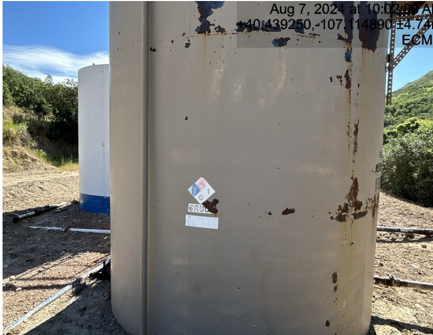
1 beeman tank in separate battery not labeled properly
