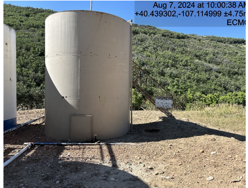
1 beeman tank in separate battery not labeled properly
