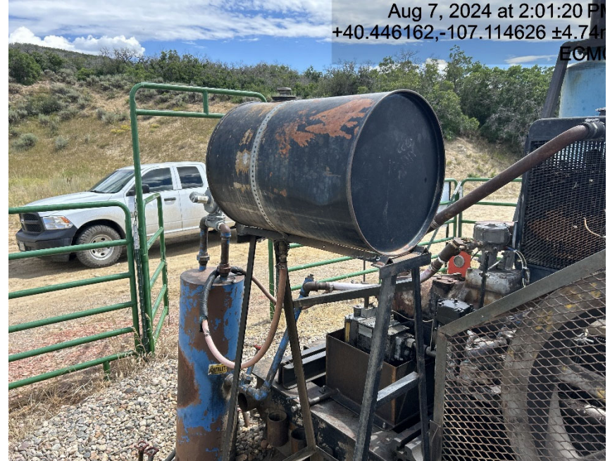
Unknown contents / no secondary containment
