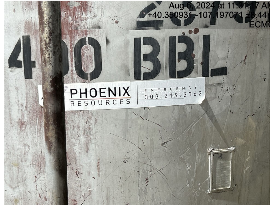
Tank signage lacking information
