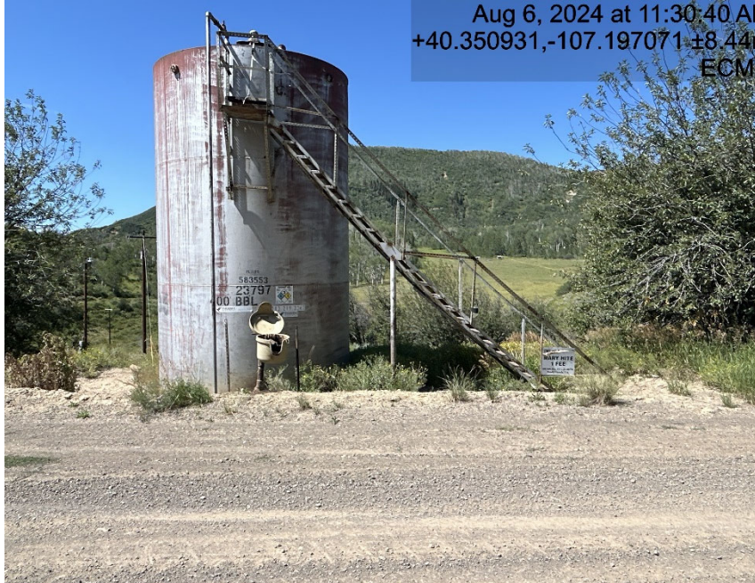
Tank battery signage lacking information
