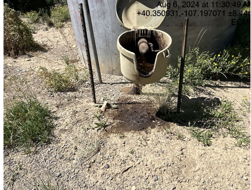
Load out bucket over flowing and stained soils under it
