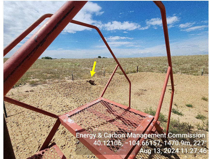
Photo 4: hole in berm
