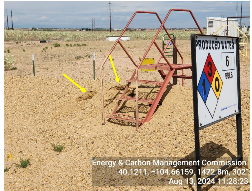
Photo 6: holes in berm
