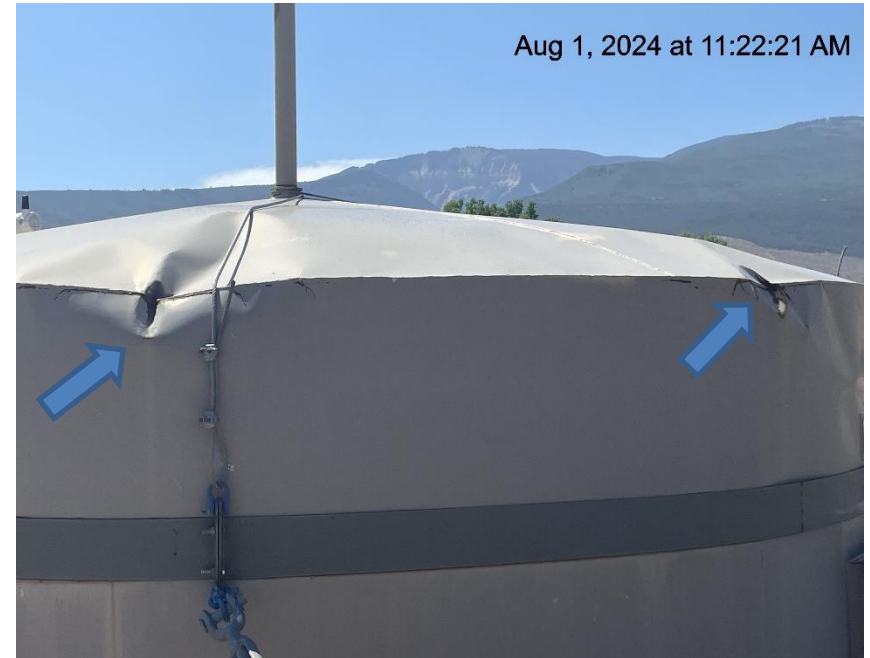
Photo # 4354 Production tank damaged
