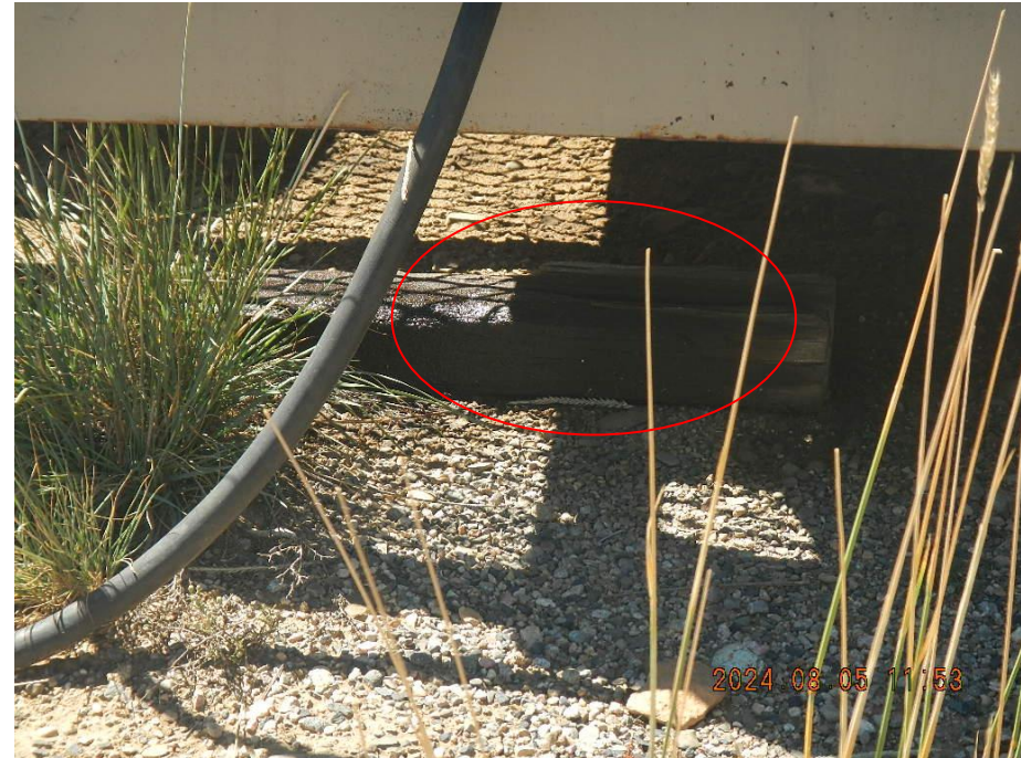
Photo 6. Lube oil on the ground and timber beneath generator.
