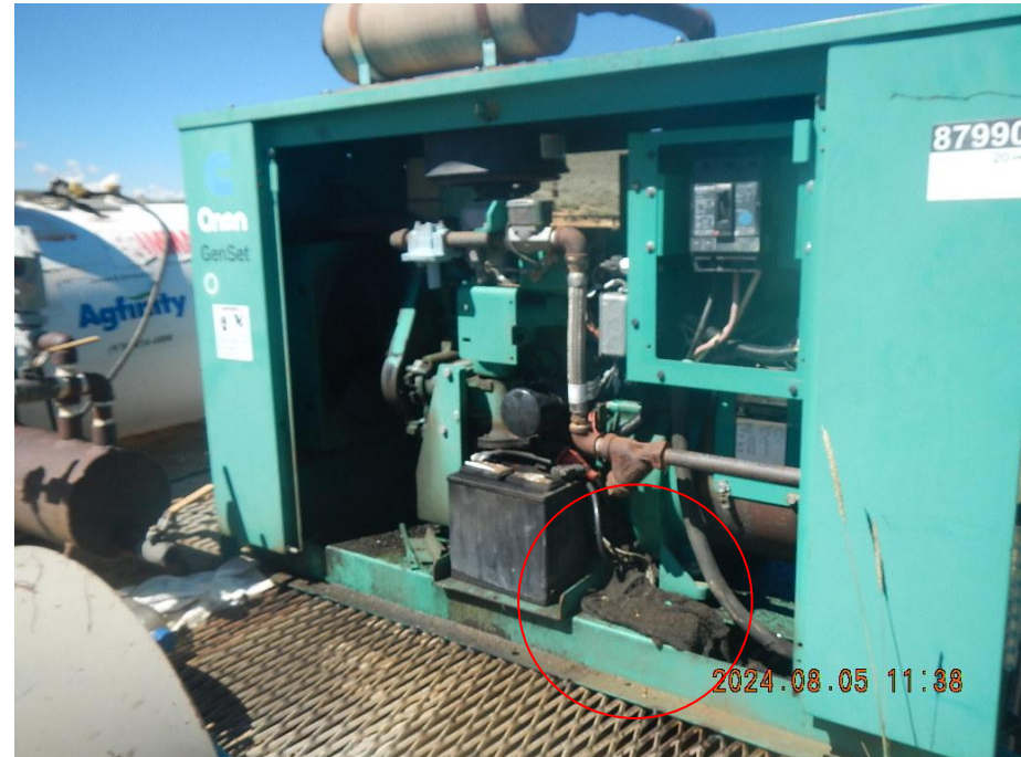
Photo 4. Oily rag and oil inside of generator cabinet.
