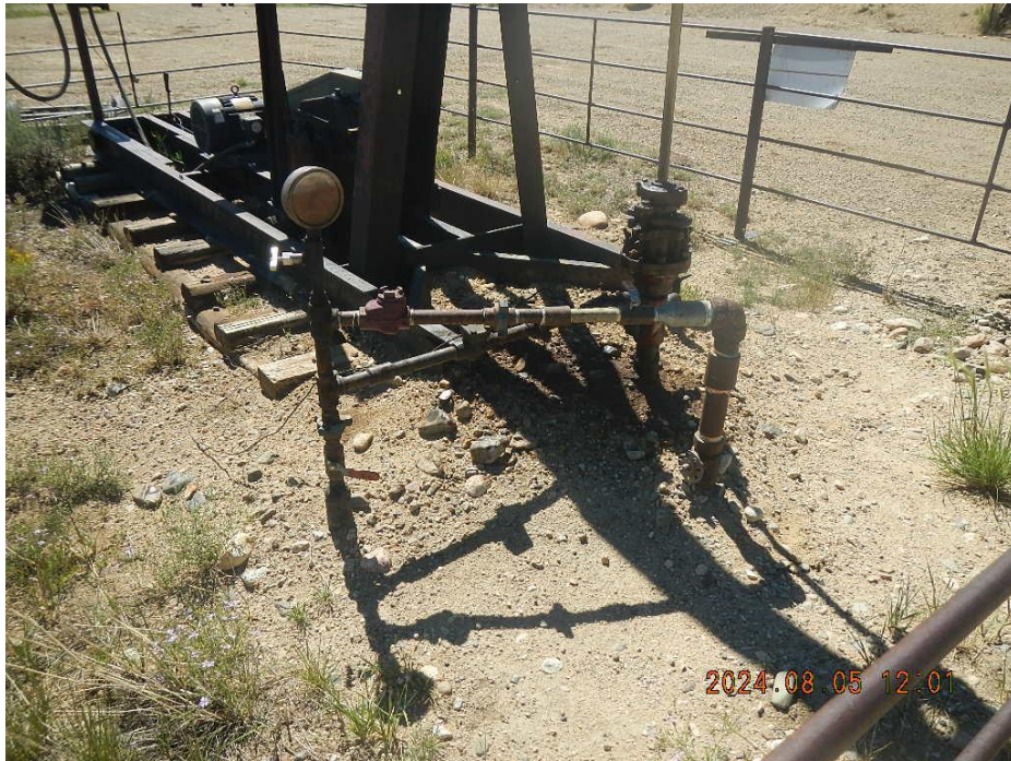
Photo 7. Oil staining on the ground at well head.
