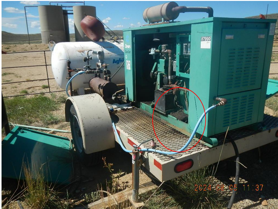
Photo 3. Oily rag and oil inside of generator cabinet.
