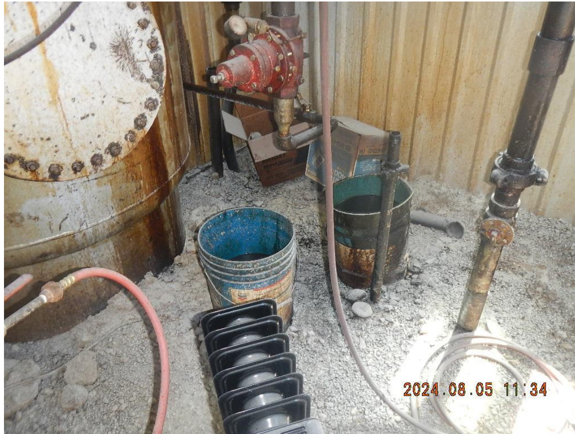
Photo 2. Improper storage of E&P Waste in 5-gallon buckets (Rule 905.a.(1)).
