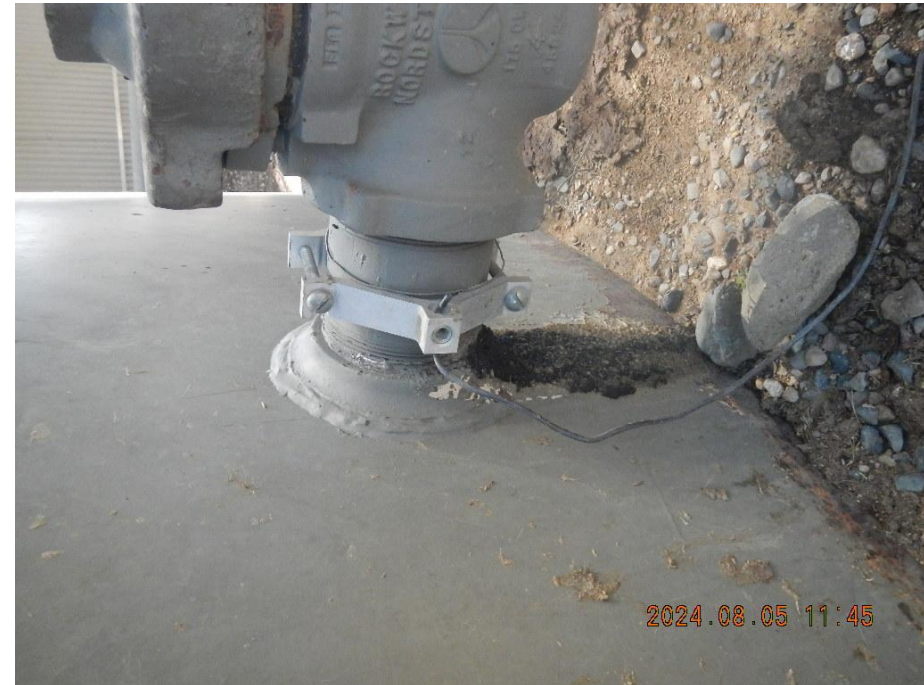
Photo 16. Staining on tank beneath threaded nipple to valve.
