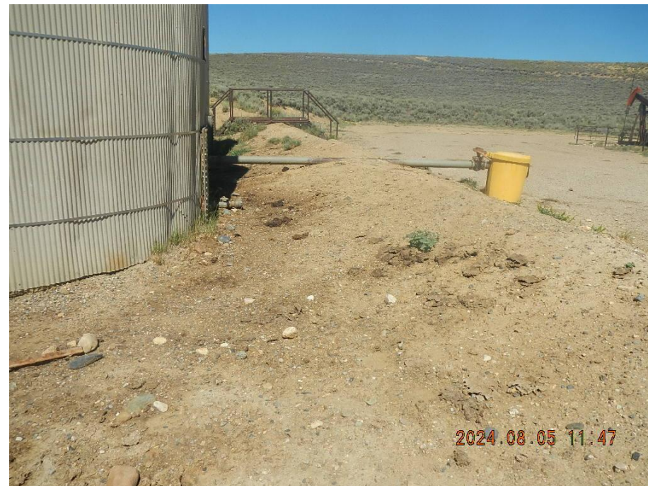
Photo 14. Evidence of livestock on tank battery berms.
