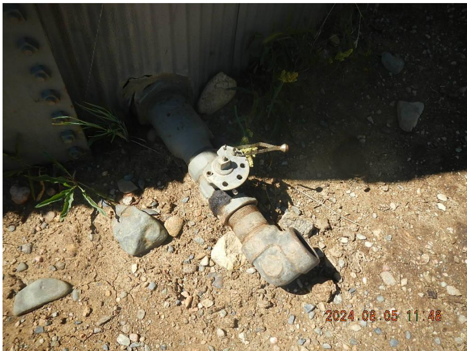
Photo 21. Oil weeping from valve on Tank # 157271_111716
