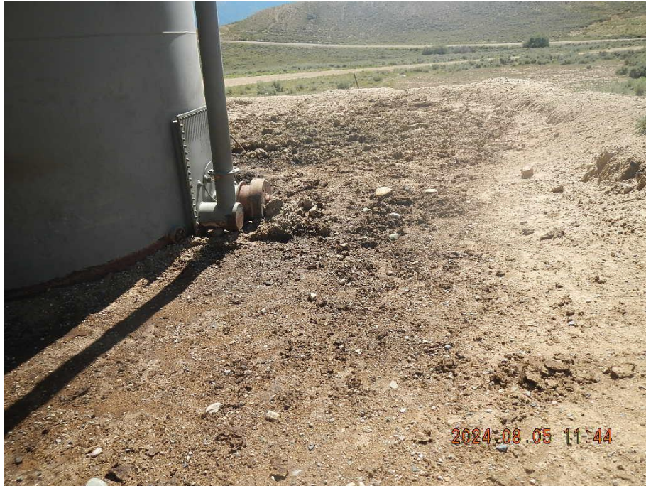
Photo 17. Evidence of livestock and insufficient berm.
