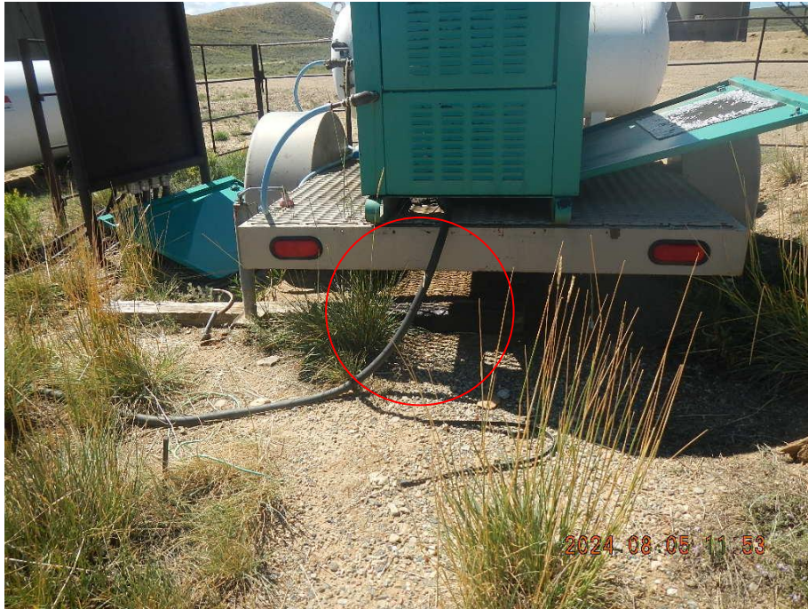
Photo 5. Lube oil staining on ground beneath generator.
