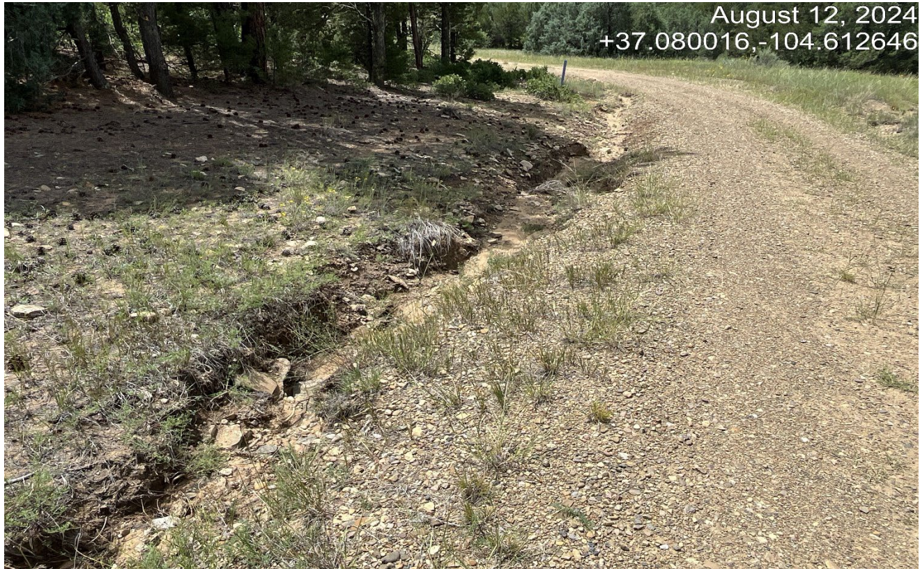
Photo 1. Facing southwest along the access road. There is erosion along the roadside that will need BMP's.
