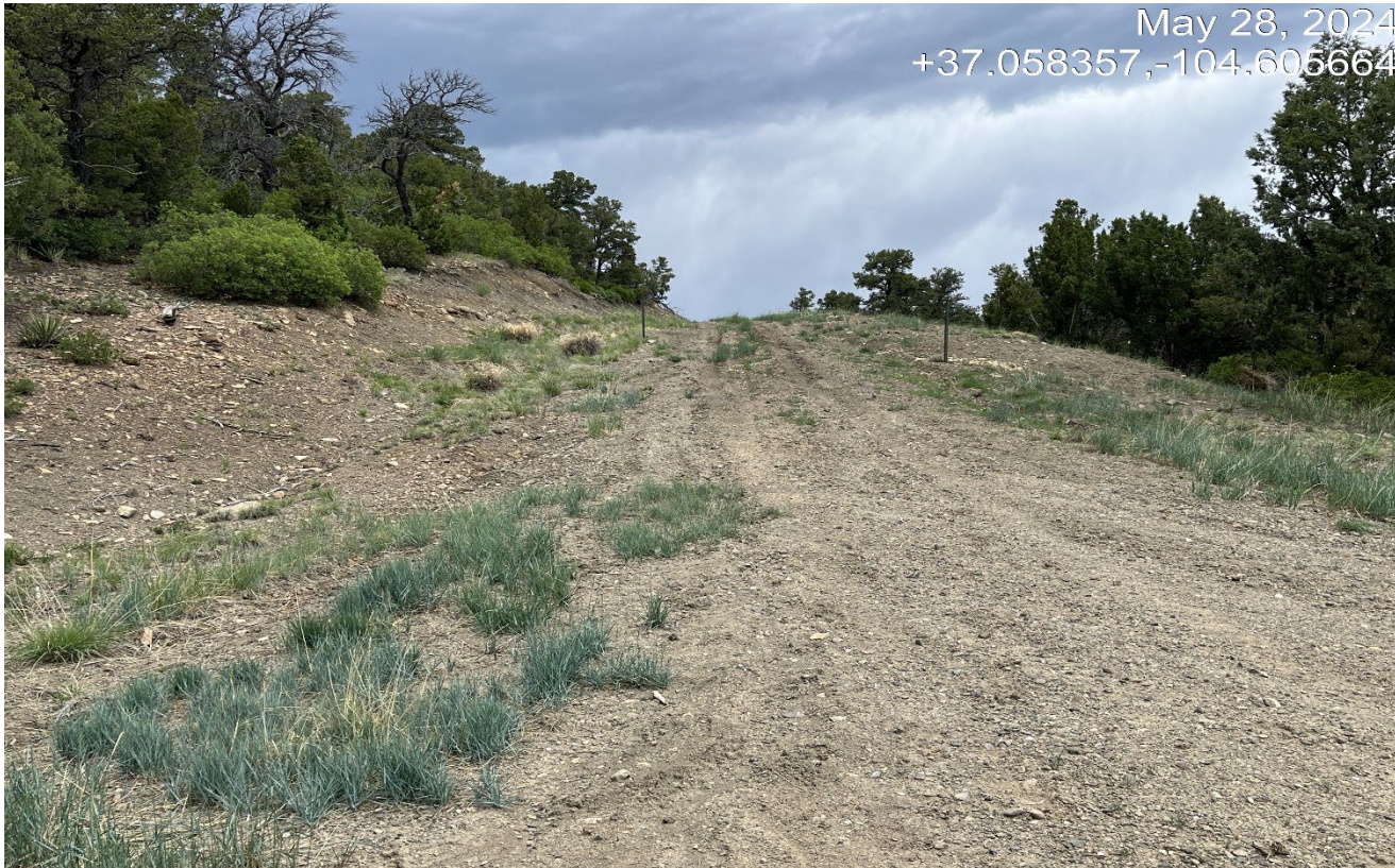
Photo 1. Facing northwest at the beginning of the access road that remains by approved variance.
