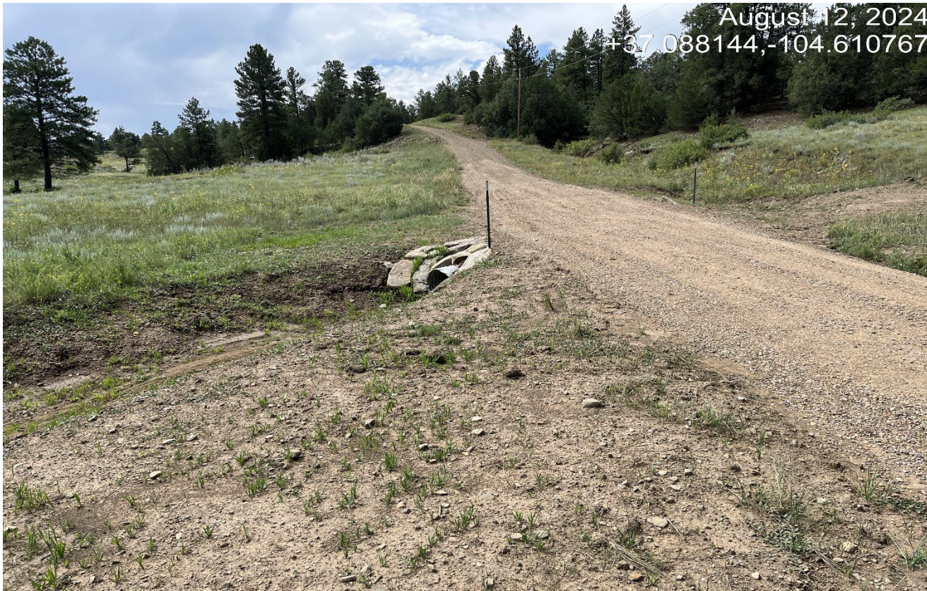
Photo 2. Facing south along the access road. This culvert has been replaced.
