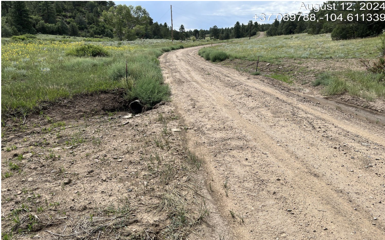
Photo 1. Facing south along the access road. The road and culvert have been repaired.
