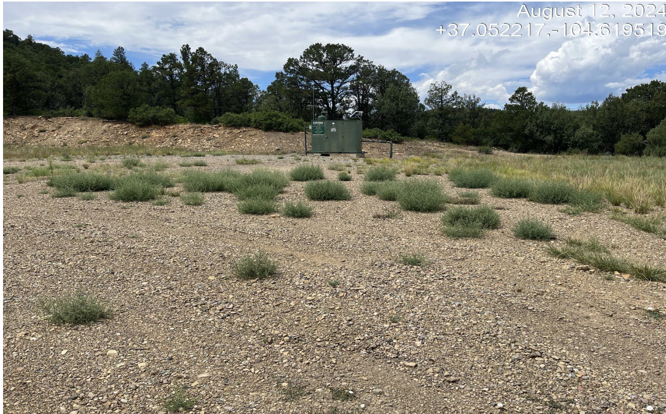
Photo 2. Facing southwest at the location. Well sign is posted at meter shed..
