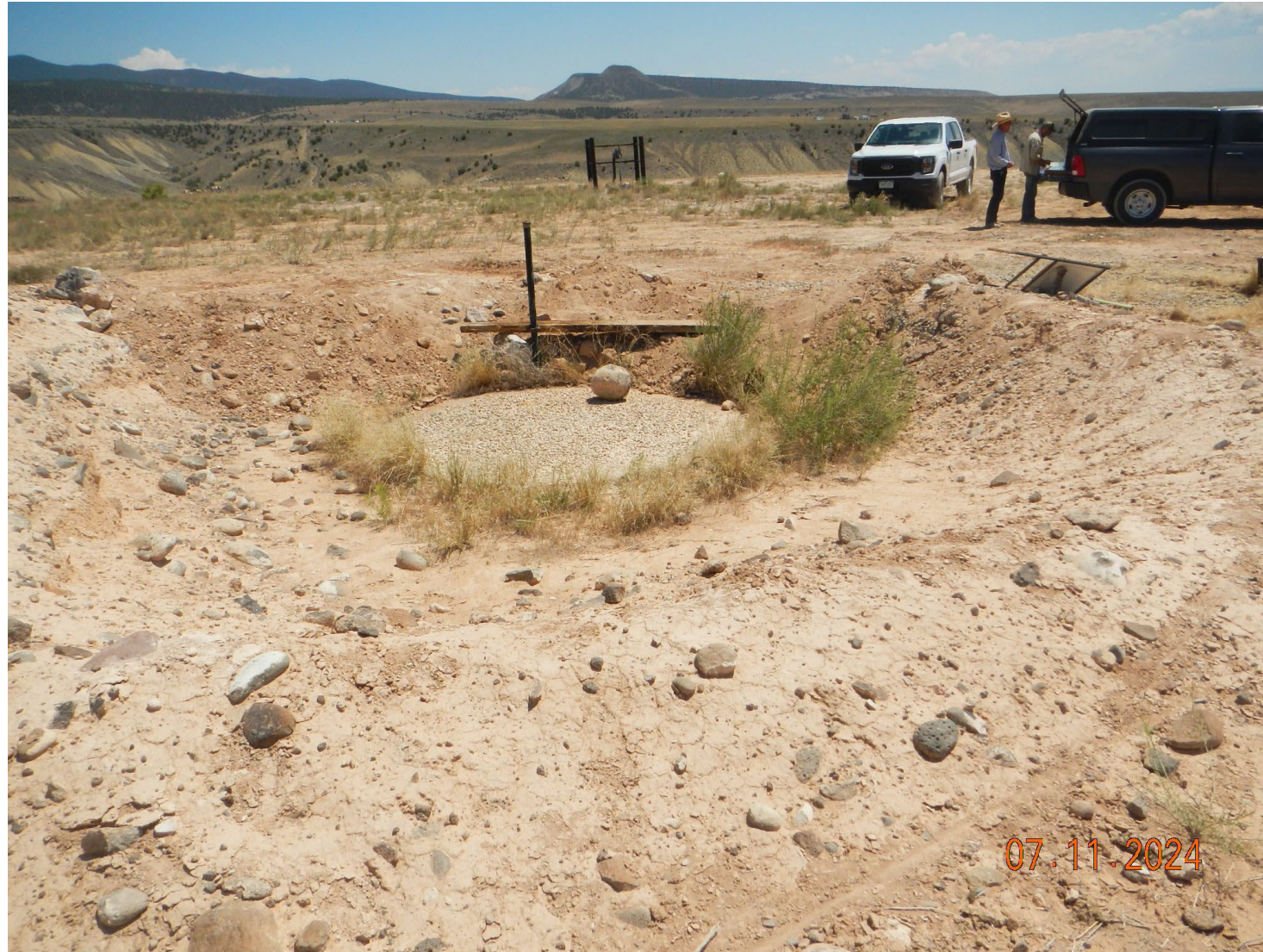
• Photo 2 – Doty 1-1 (OWP) tank battery area
