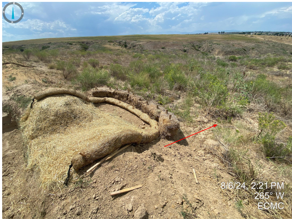
Photos 17 & 18. Taken near the northern portion of the construction area. Evidence of off location sediment transport observed near one of the sediment traps.
