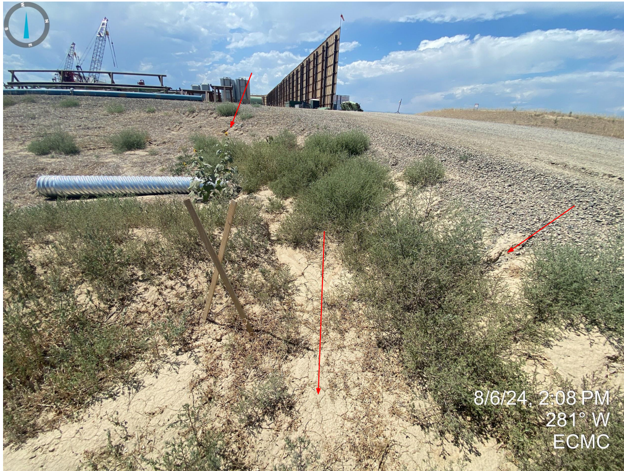
Photo 7. Taken near the location entrance. Photo illustrates undesirable vegetation and sediment discharge and erosion degradation (riling) near the culvert crossing.
