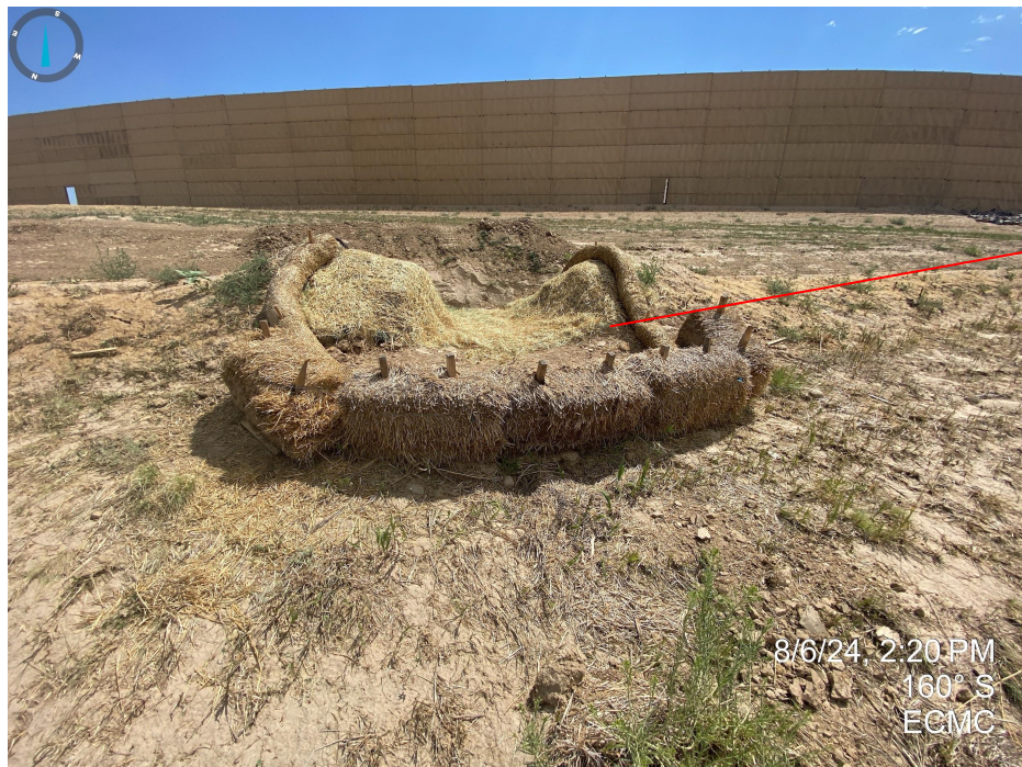
Photo 15 & 16. Taken near the northern portion of the construction area. Evidence of off location sediment transport observed near one of the sediment traps.
