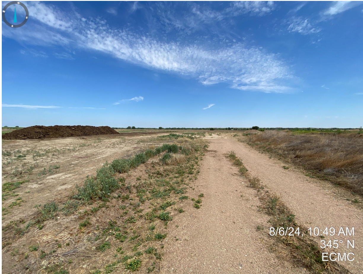
Photo 1. Taken south of the former tank battery and well location. Photo illustrates the access road does not appear to have been reclaimed with road base still present.
