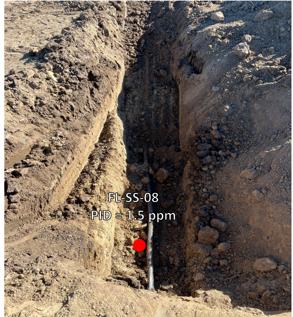
Looking east at bellhole/cut point for removal
