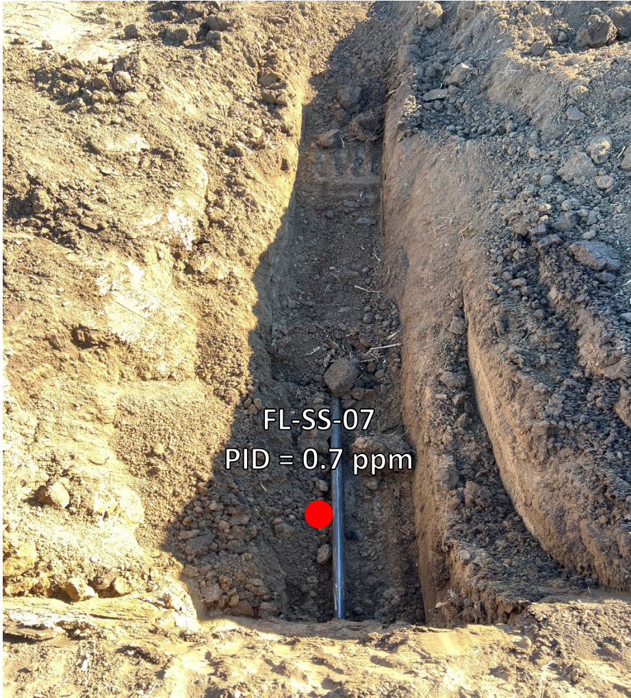
Looking east at bellhole/cut point for removal
