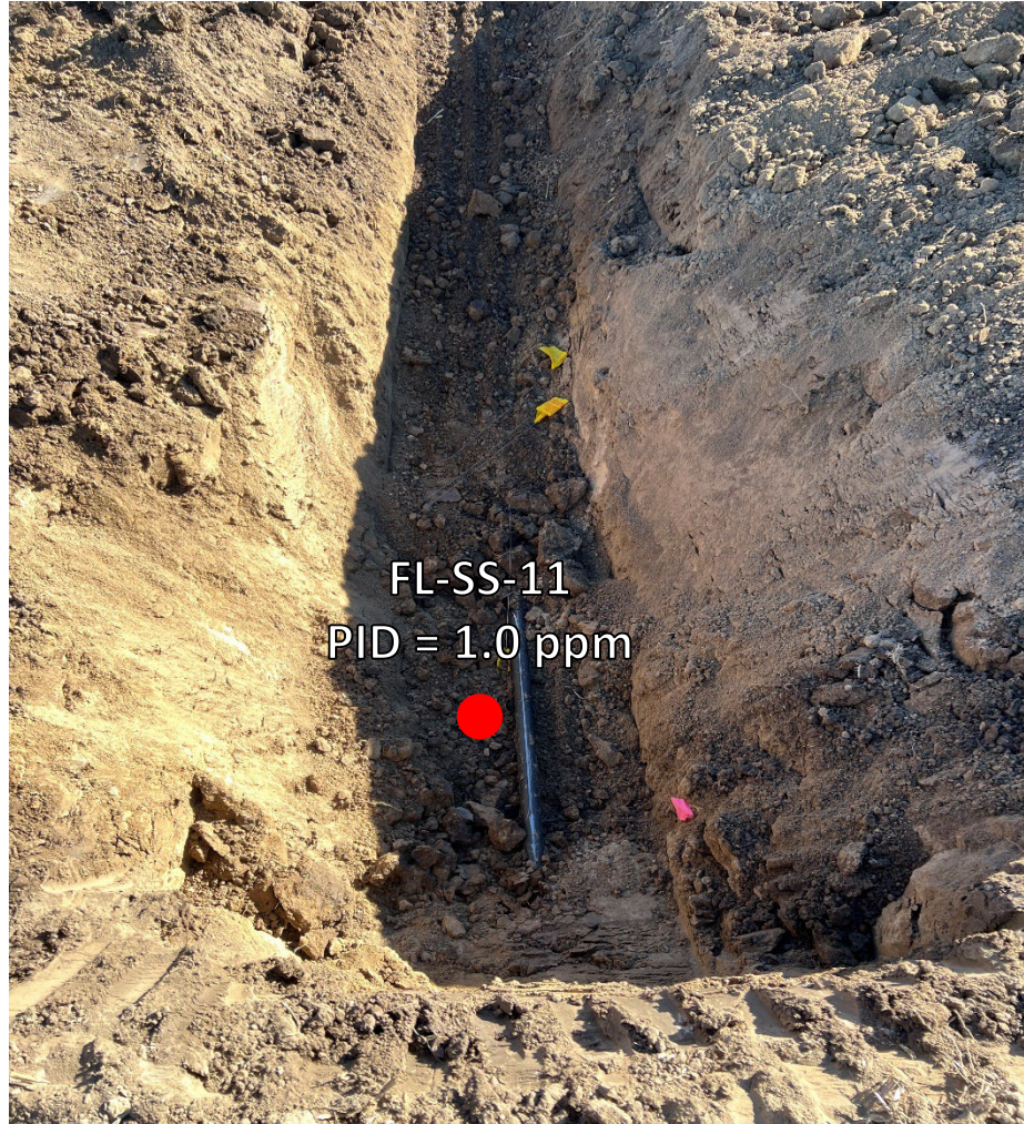
Looking east at bellhole/cut point for removal
