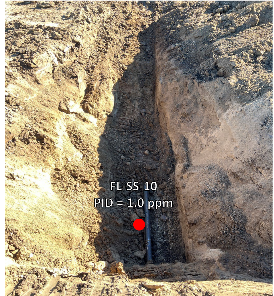
Looking east at bellhole/cut point for removal
