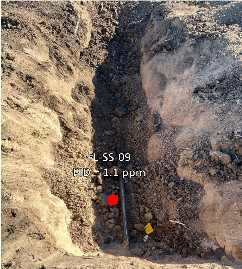
Looking east at bellhole/cut point for removal
