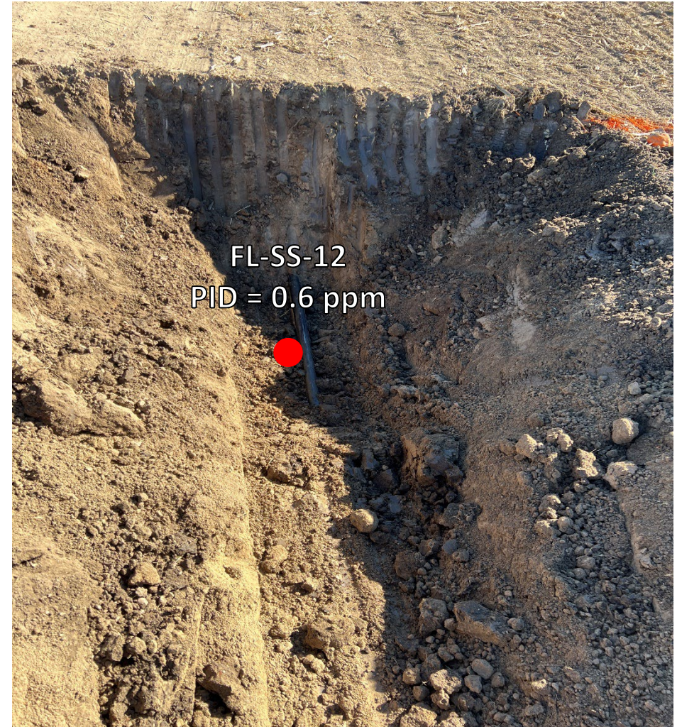
Looking east at cut point of abandonment
