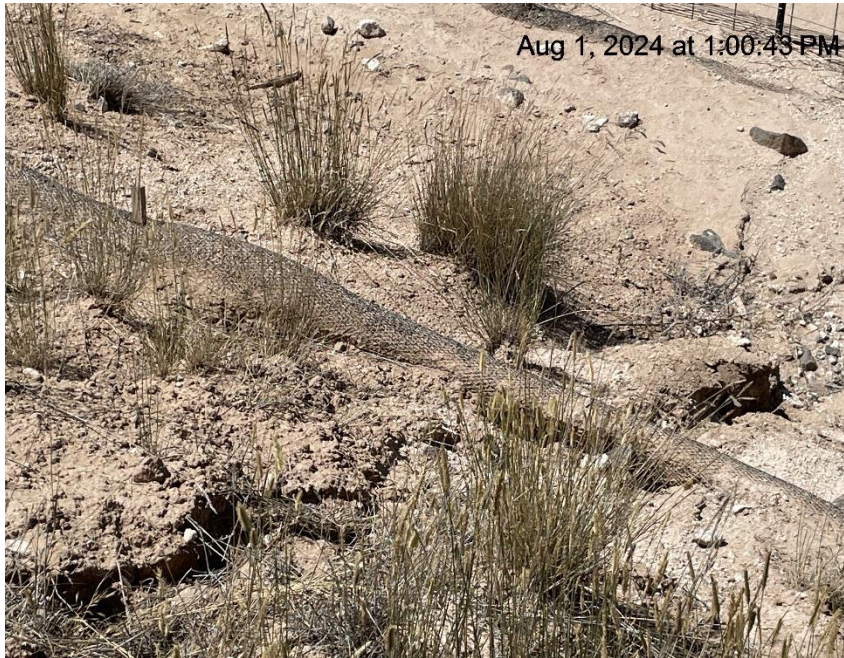
Photo # 4443 Erosion & transport of sediment/wattles need maintenance
