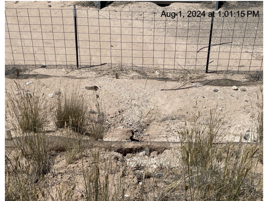
Photo # 4444 Erosion & transport of sediment/wattles need maintenance
