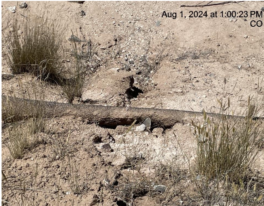
Photo # 4441 Erosion & transport of sediment/wattles need maintenance
