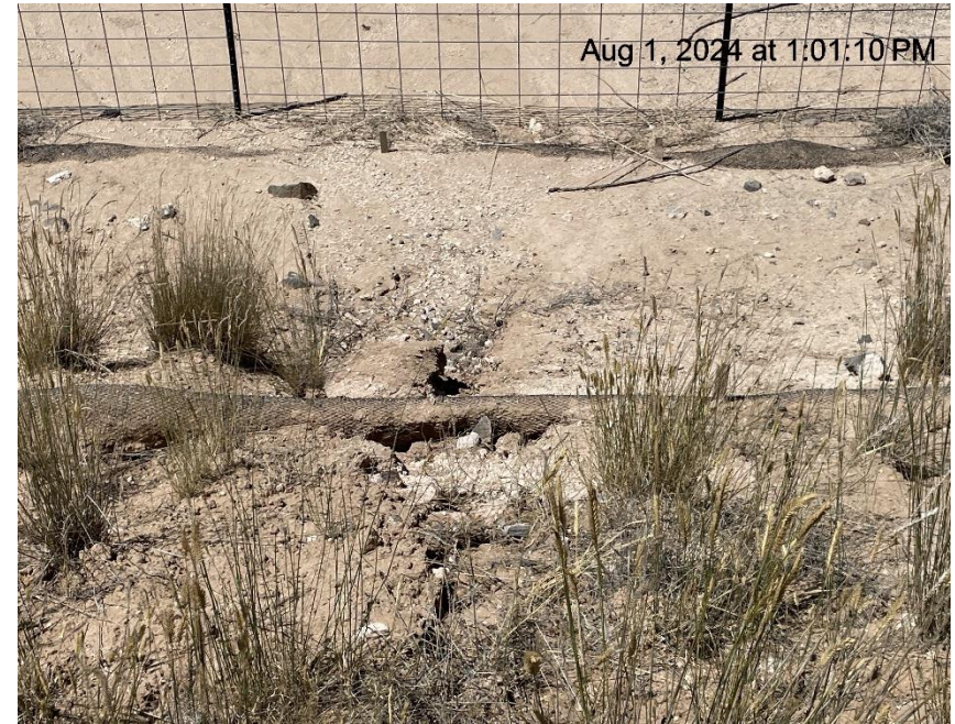
Photo # 4442 Erosion & transport of sediment/wattles need maintenance
