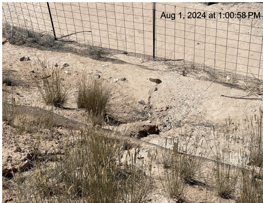
Photo # 4445 Erosion & transport of sediment/wattles need maintenance
