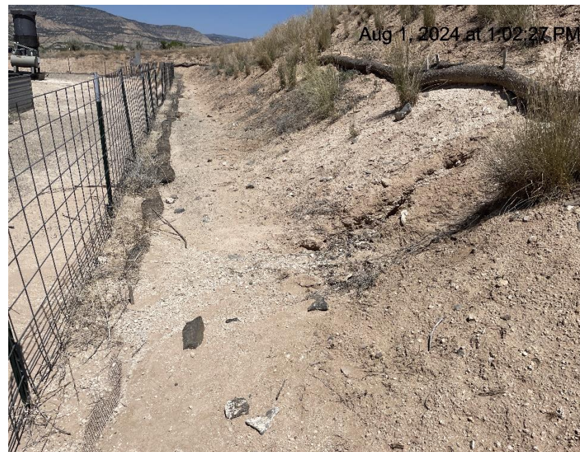
Photo # 4446 Erosion & transport of sediment/wattles need maintenance
