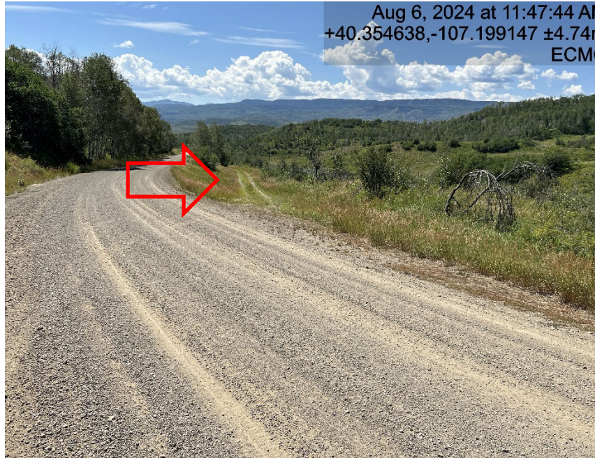
Access road covered with weeds
