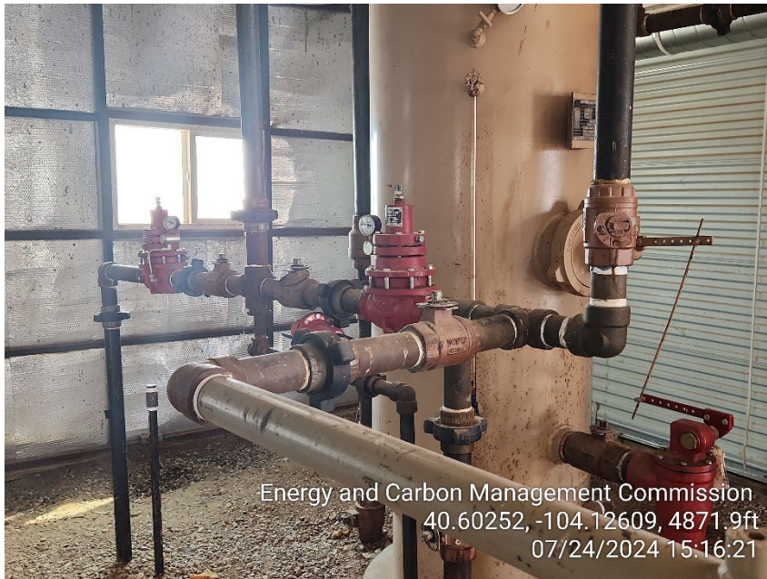
Photo 13 – Flare Line Valves appear to be in the open position
