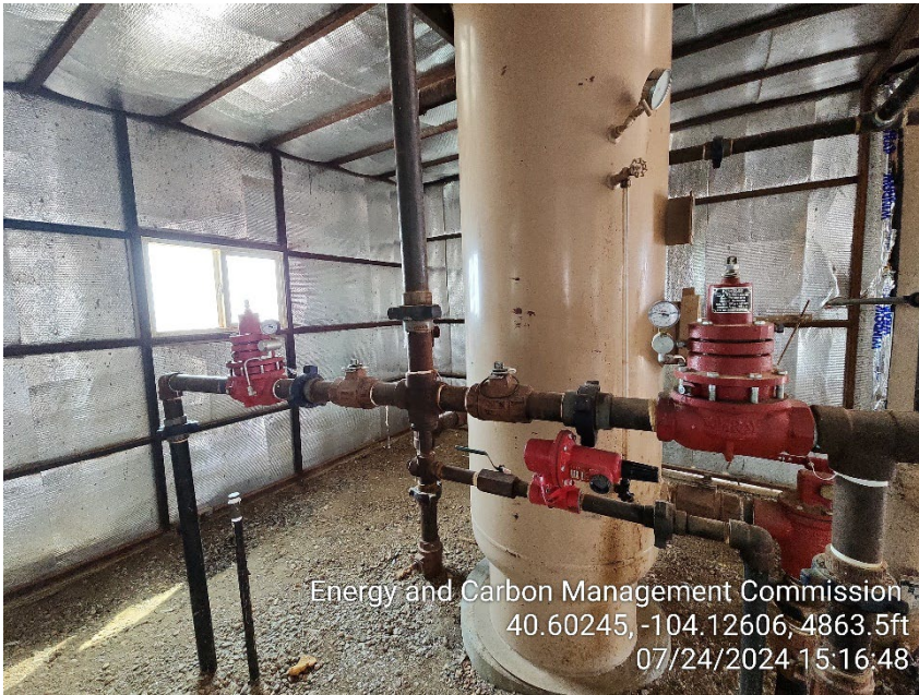
Photo 15 – Flare Line Valves appear to be in the open position
