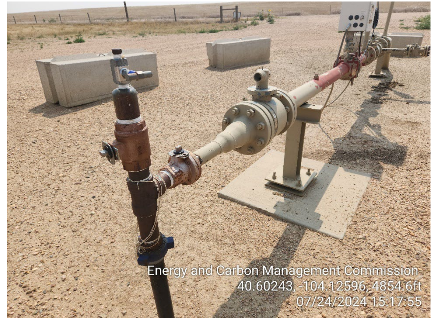
Photo 16 – Sales Line Valve appears to be in the open position
