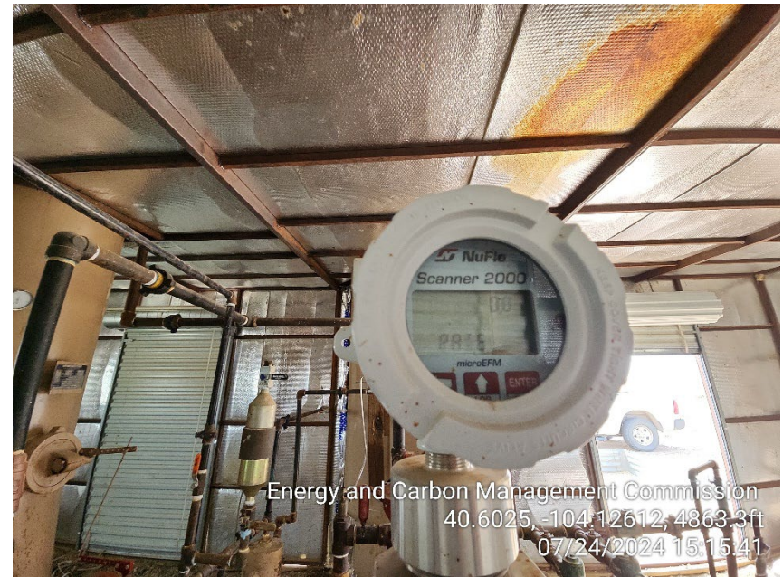
Photo 10 – Flare Gas Meter – Rate
