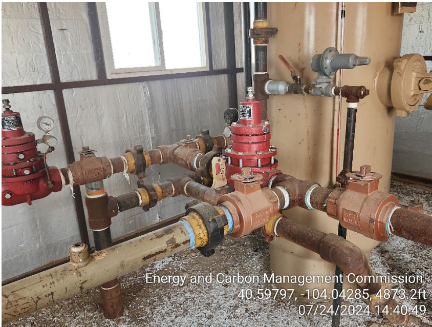
Photo 11 – Sales Line Valve and Flare Line Valves appear to be in the open position
