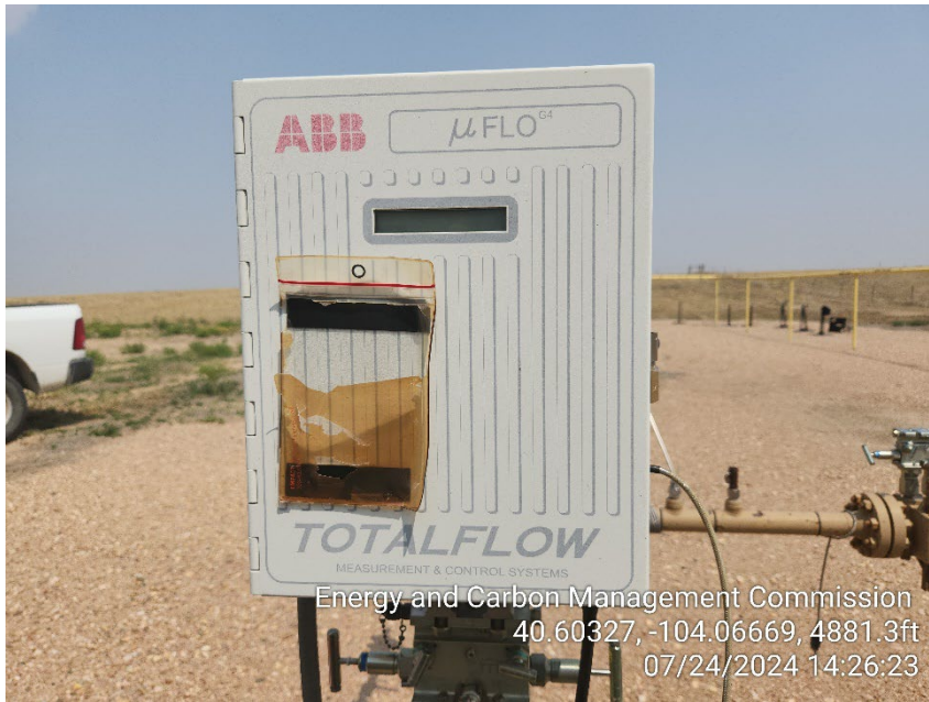
Photo 9 – Gas Sales Meter appears to be powered off
