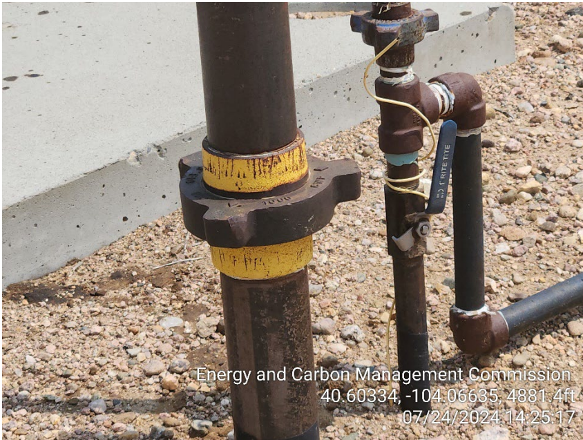
Photo 5 – Pilot Supply Valve appears to be in open position
