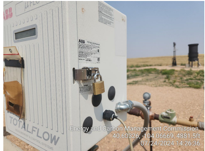
Photo 10 – Gas Sales Meter – Locked Out
