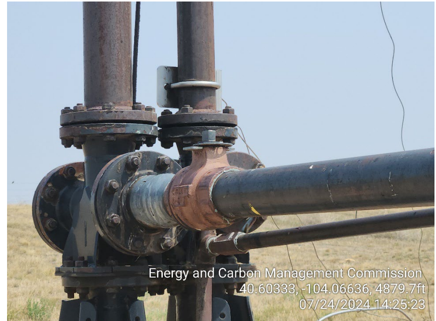
Photo 6 – Inlet Valve to Flare appears to be in open position
