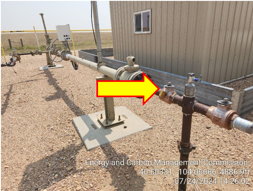
Photo 7 – Gas Sales Line and Meter – Locked Out
