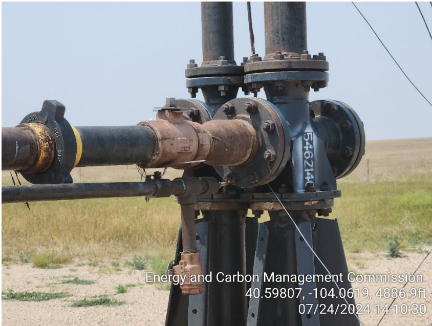
Photo 9 – Pilot Valve appears to in open position
