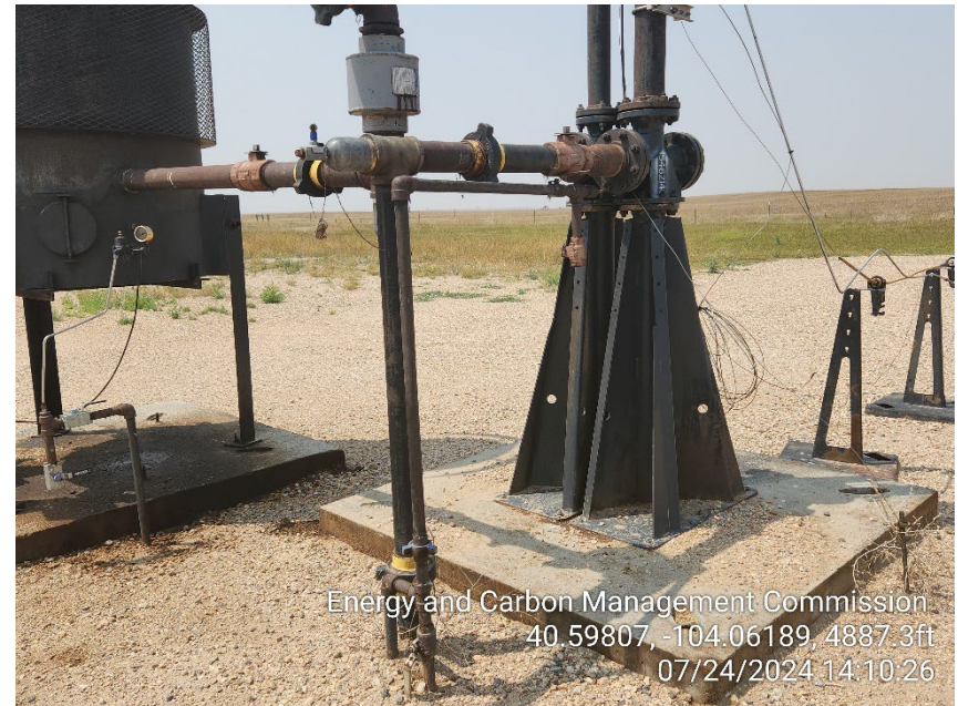
Photo 8 – Inlet Valves to Flare appear to be in open position
