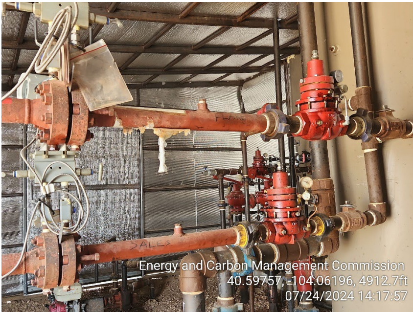
Photo 23 – Flare and Sales Meters inside Treater House
