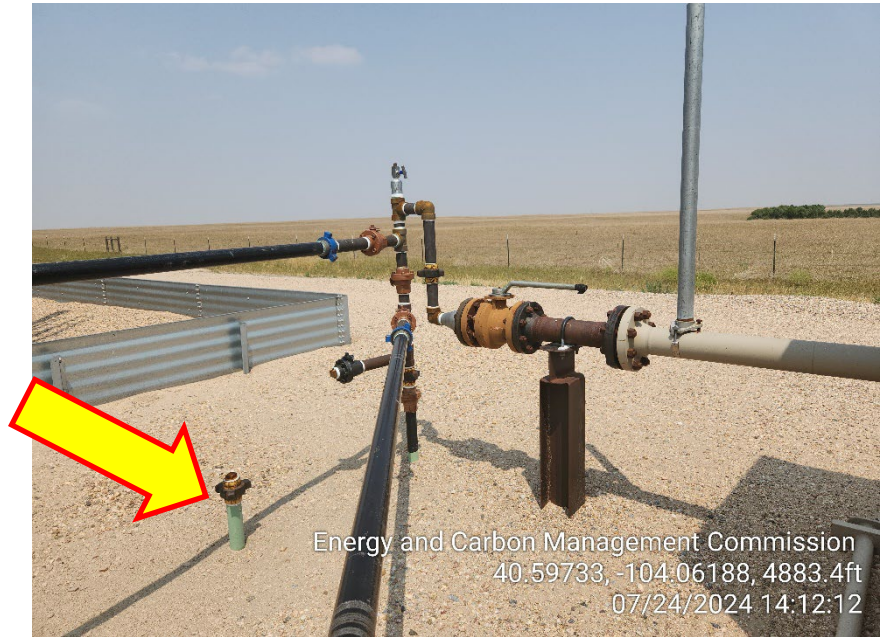
Photo 14 – Sales Line – Unmarked Riser
