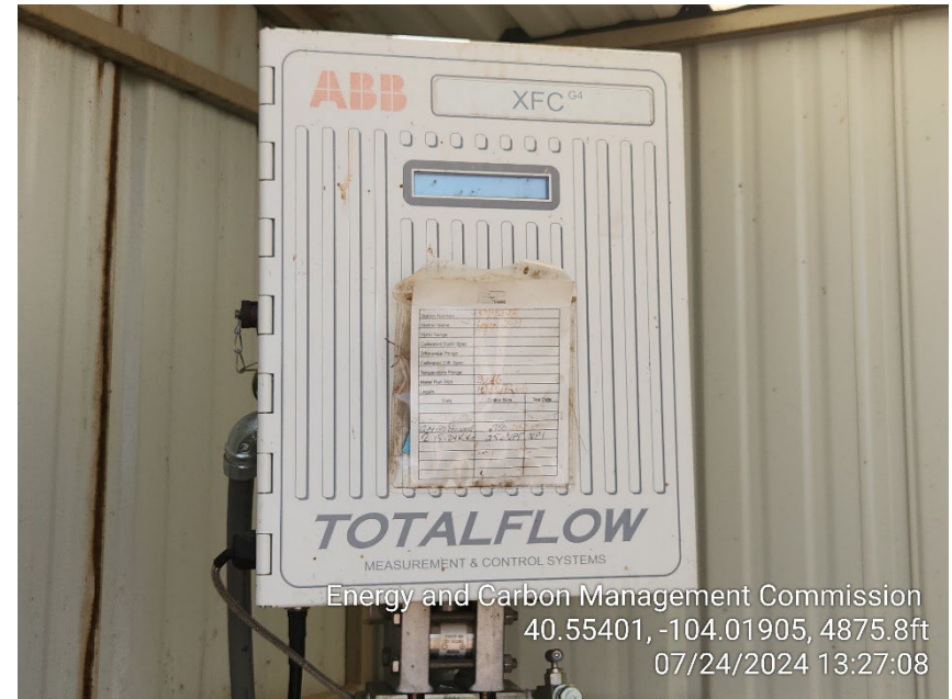
Photo 6 – Sales Meter appears to be powered off
