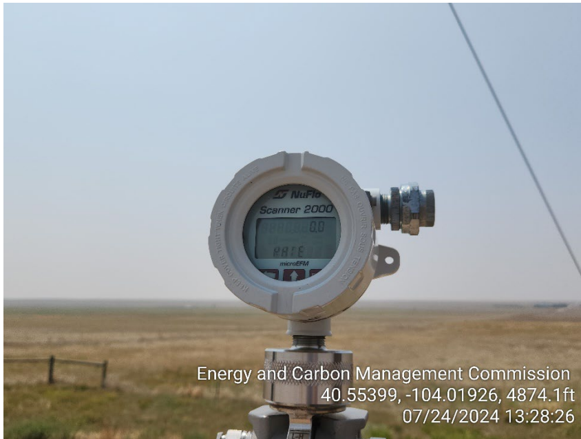
Photo 11 – Flare Gas Meter – Flow Rate
