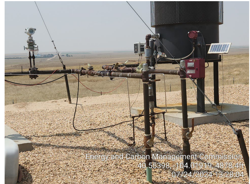
Photo 8 – ECD and Flare Gas Meter
