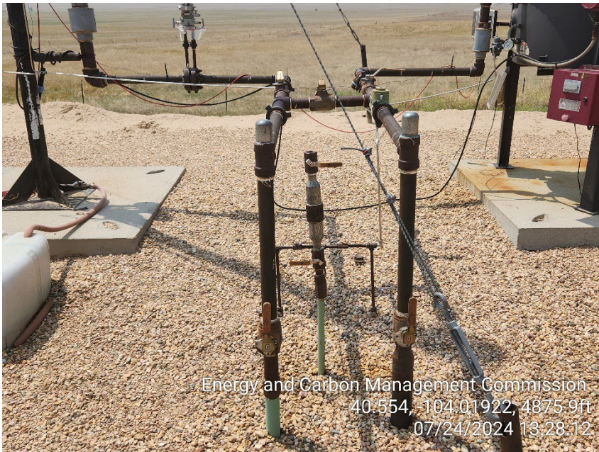
Photo 9 – Flare inlet Valves appear to be in open position
