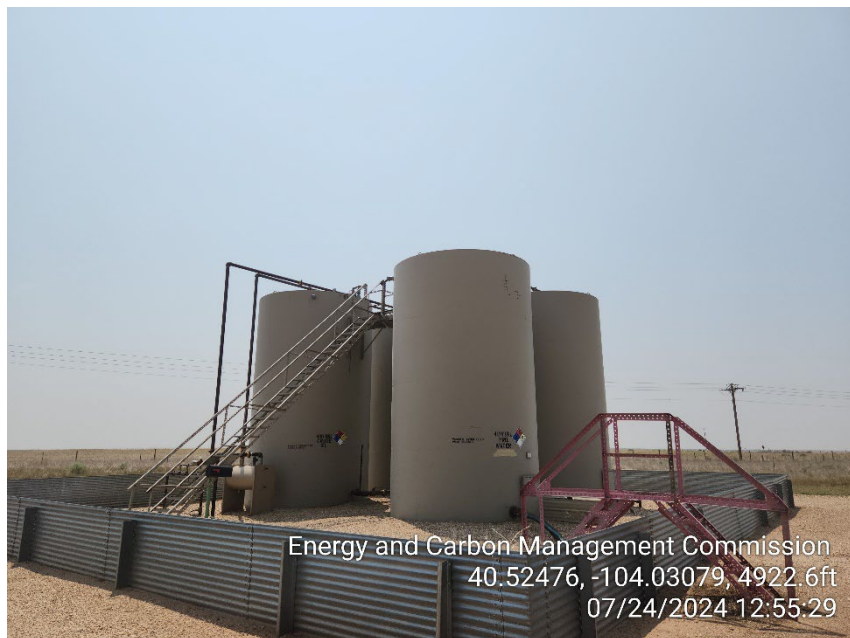
Photo 19 – Tank Battery
