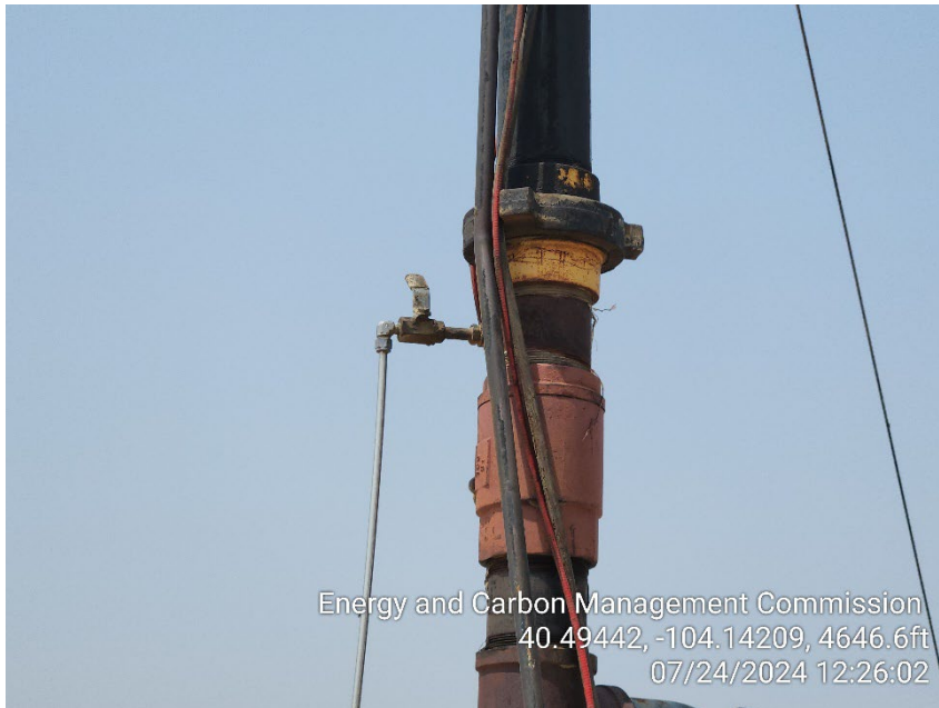
Photo 15 – Pilot to Flare appears to be in the Closed Position
