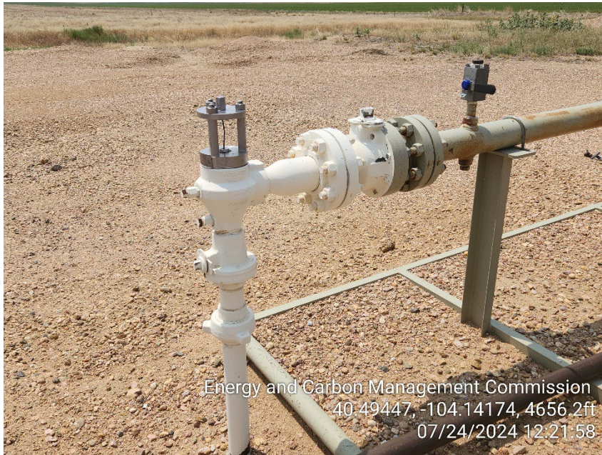
Photo 5 – Sales Line Valves appear to be in open position
