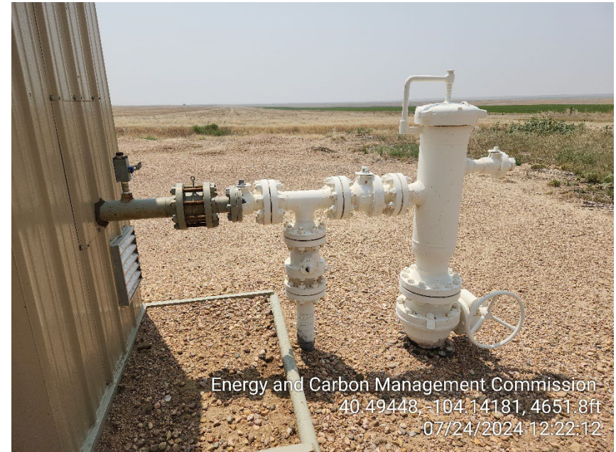
Photo 6 – Sales Line Valves appear to be in open position
