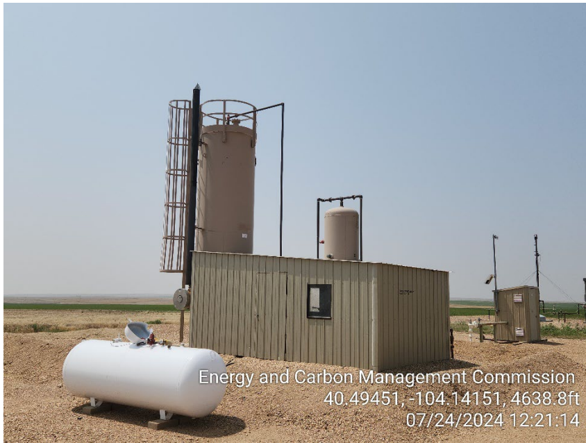
Photo 3 – Heater Treater and Propane Tank
