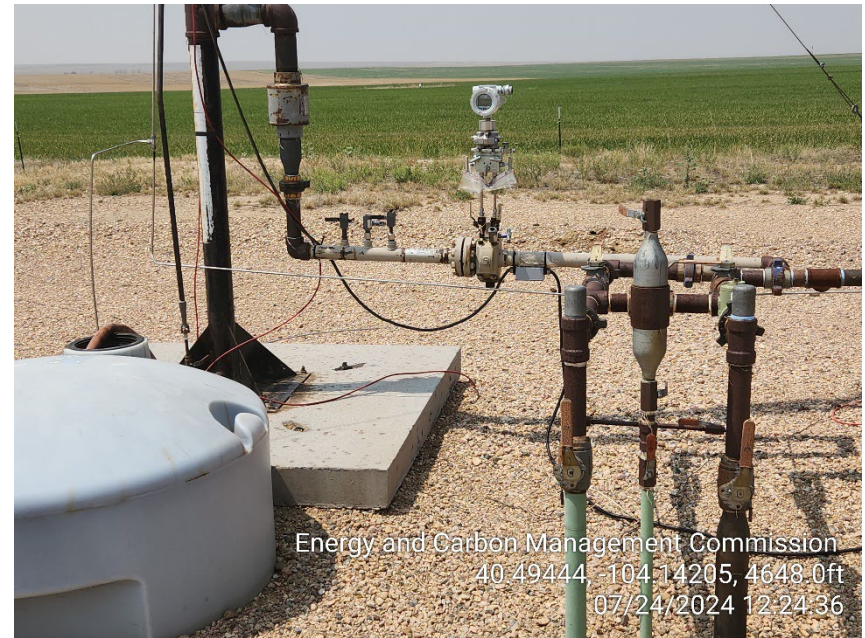
Photo 12 – Flare Gas Meter – Valves appear to be in Open position to Flare Line
