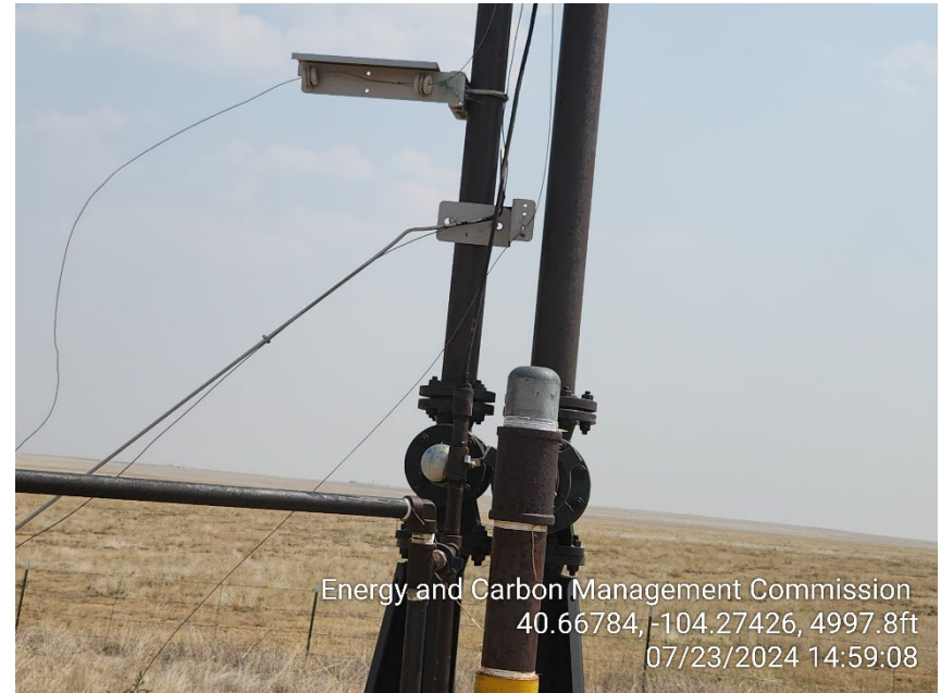
Photo 14 – Flare – Pilot supply valve open
