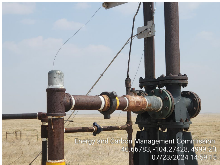
Photo 15 – Valves open to Flare
