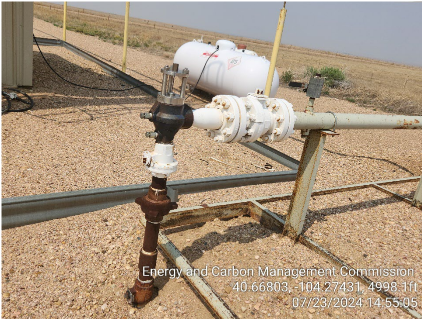
Photo 5 – Sales Line Valves in open position
