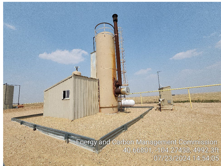
Photo 4 – Heater Treater and Gas Meter
