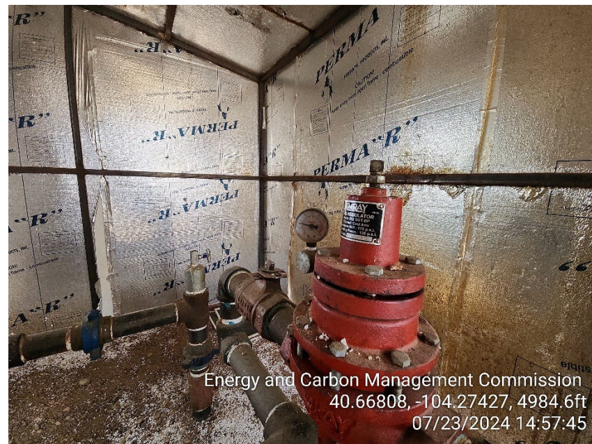
Photo 12 – Valves in Open position to Flare Line
