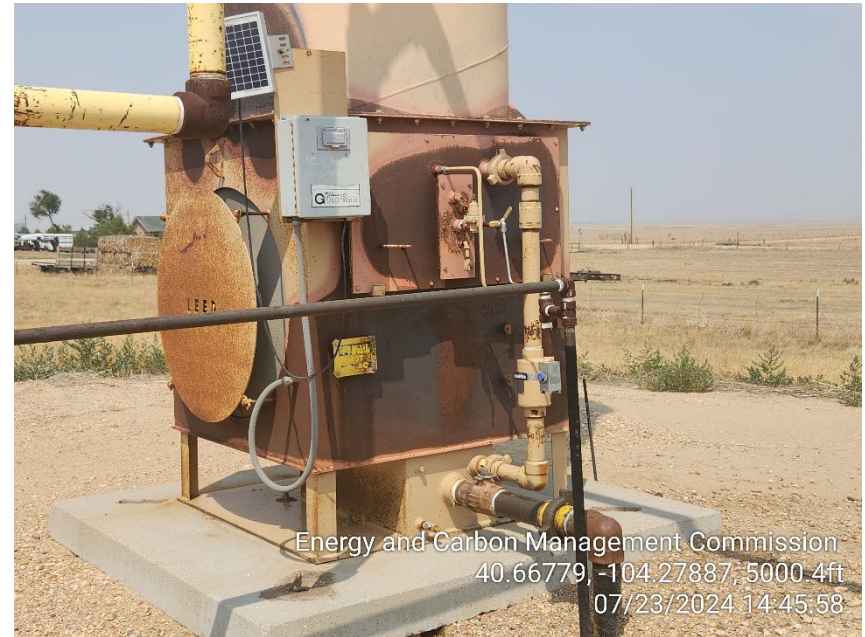
Photo 12 – Valves in Open position and Pilot Light on
