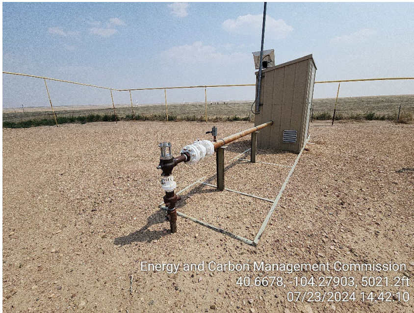
Photo 5 – Sales Line Valves in open position
