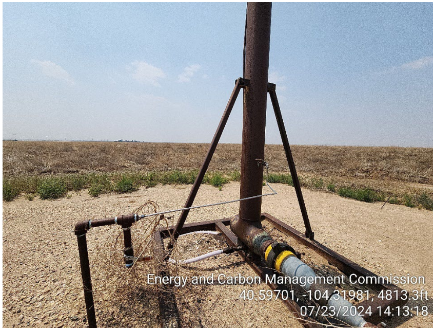
Photo 15 – Flare Valve Open on Flare Line
