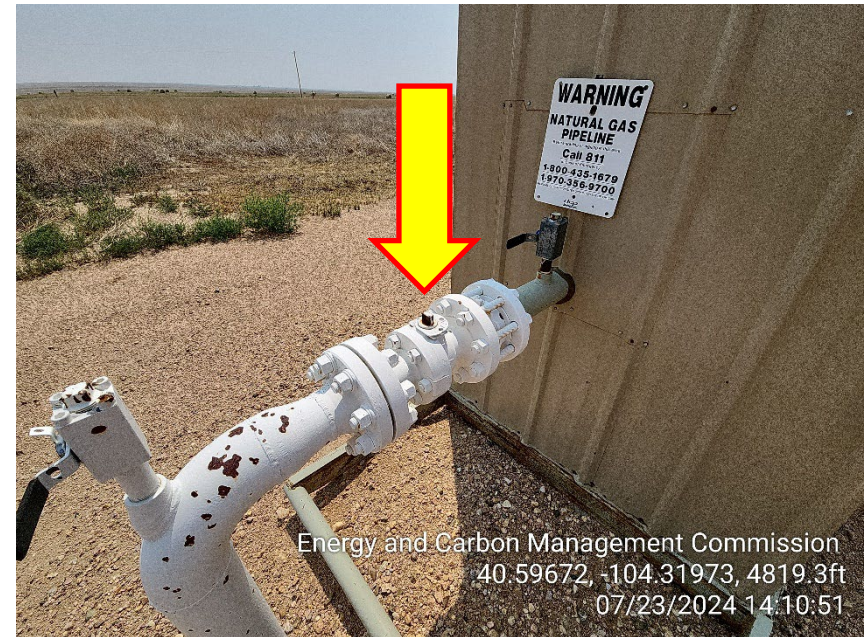
Photo 6 – Sales Line valve in the closed position
