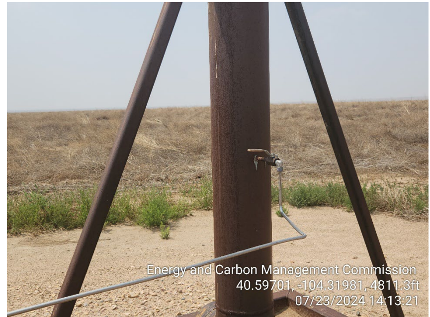
Photo 16 – Pilot Supply Valve in closed position
