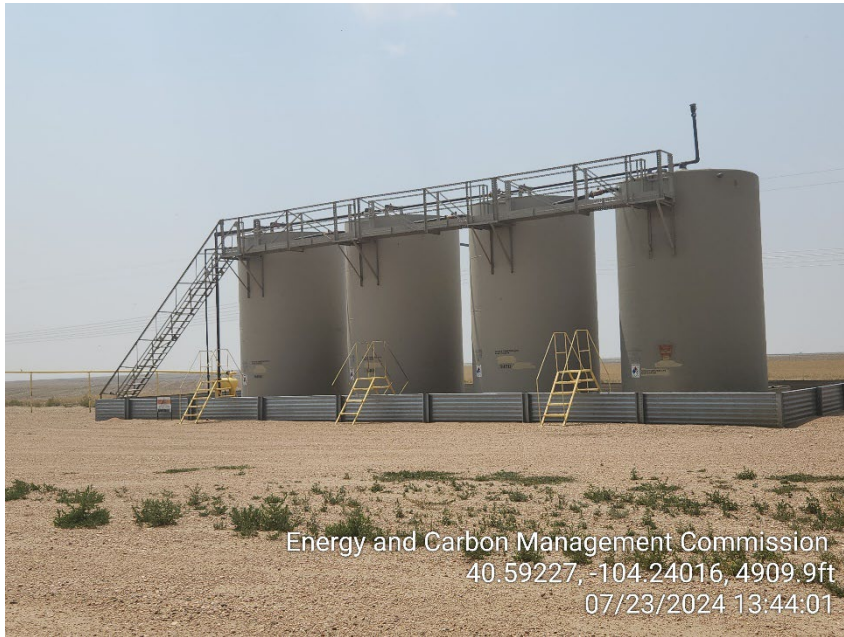
Photo 5 – Tank Battery
