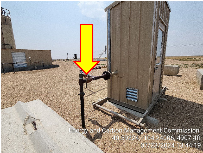
Photo 7 – Sales Line closed upstream of Meter
