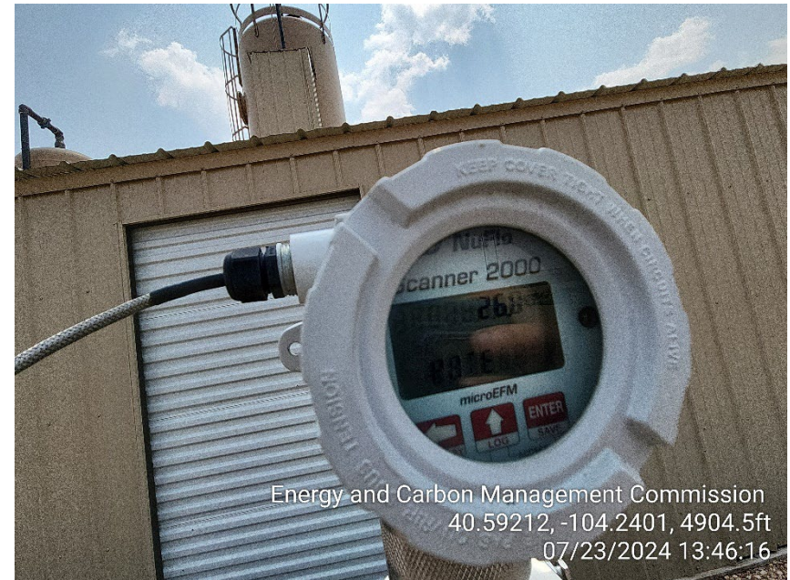
Photo 12 – Flare Gas Meter – Flow Rate
