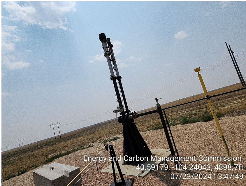
Photo 15 – Flare Valve Open on Flare Line
