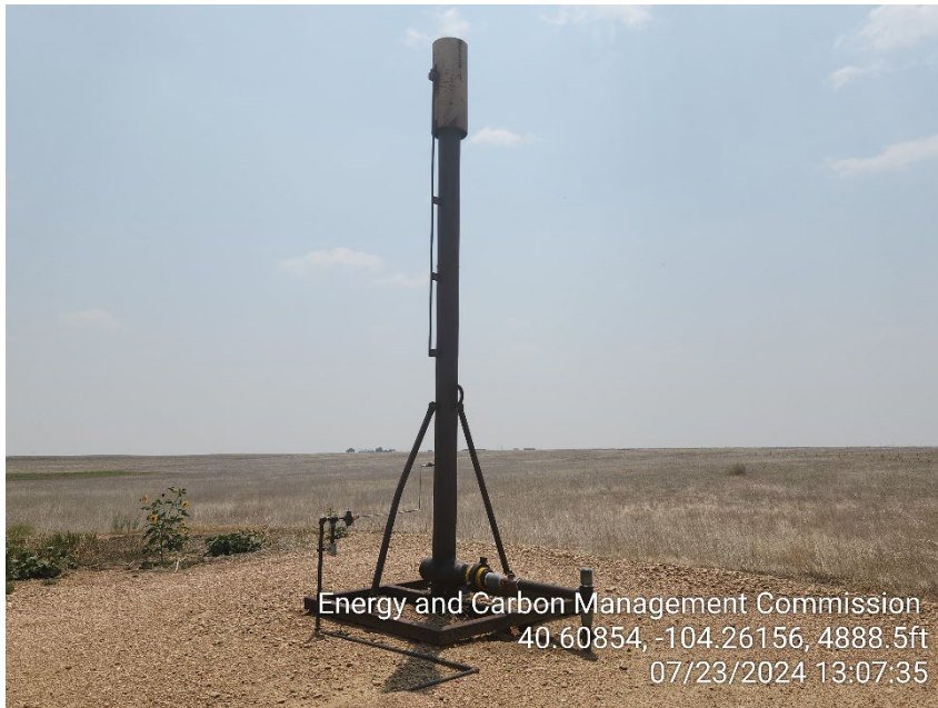
Photo 15 – Flare Valve Open on Flare Line
