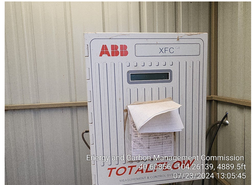
Photo 10 – Sales Meter appears to be Powered Off
