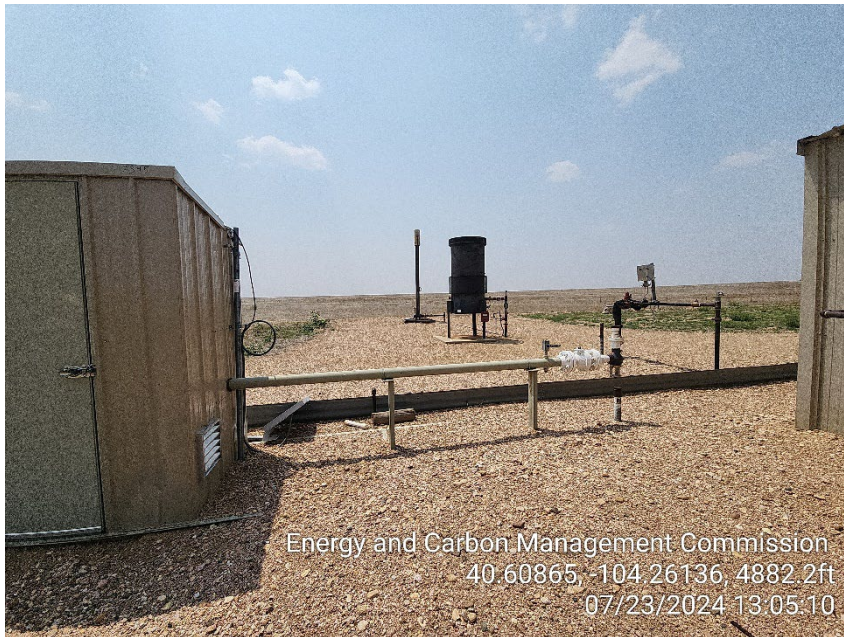
Photo 7 – Gas Meter, ECD and Flare
