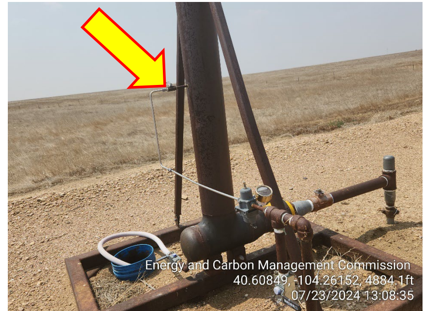
Photo 18 – Supply line to Flare in Closed position
