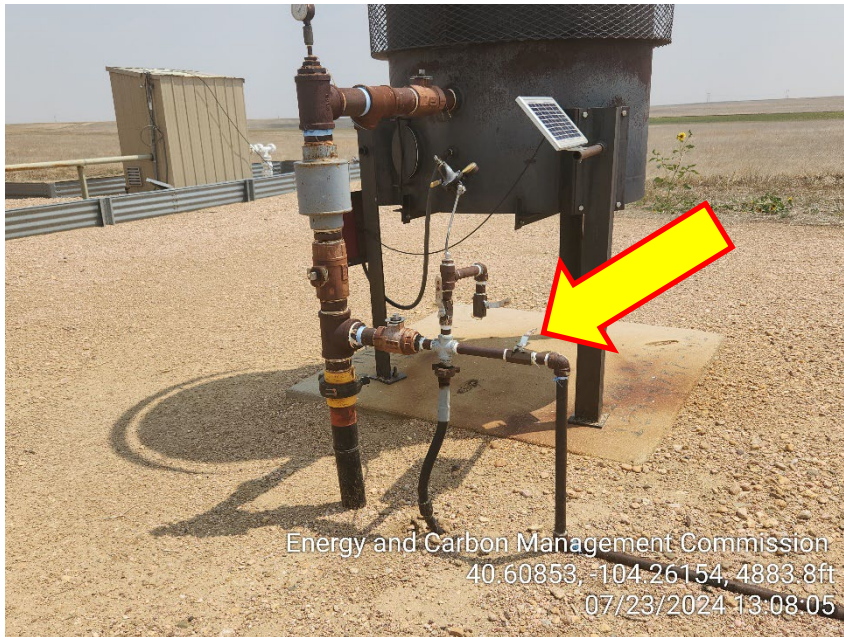
Photo 17 – ECD – 1” Supply line to Flare in Closed position
