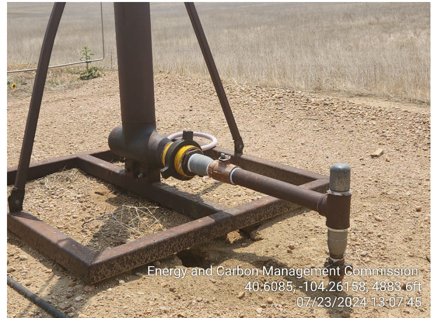
Photo 16 – Valve Open on Flare Line
