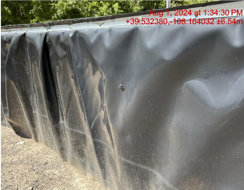
Holes in containment liner - Photo #03933
