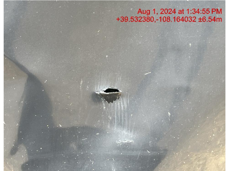
Holes in containment liner - Photo #03934
