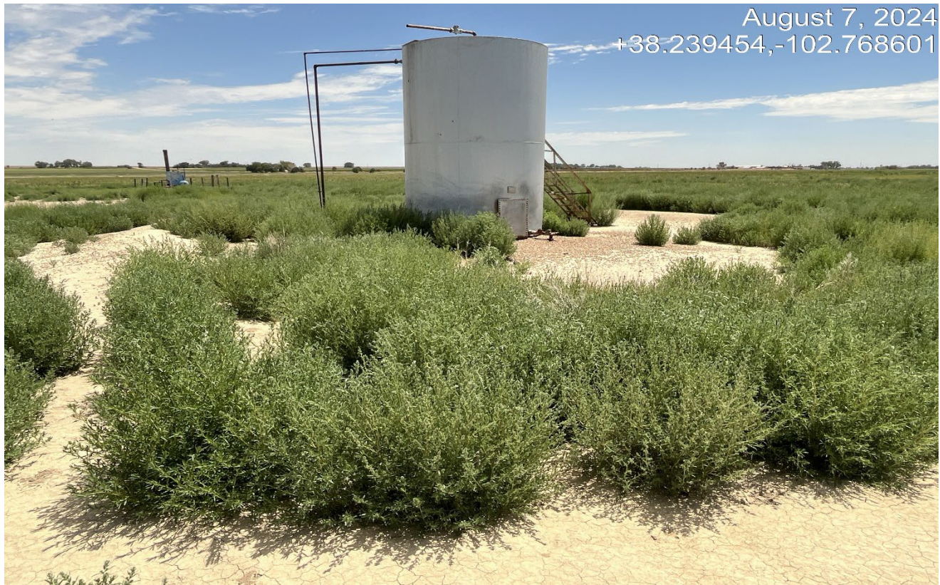
Photo 3. The secondary containment around the tank is insufficient to contain a spill .
