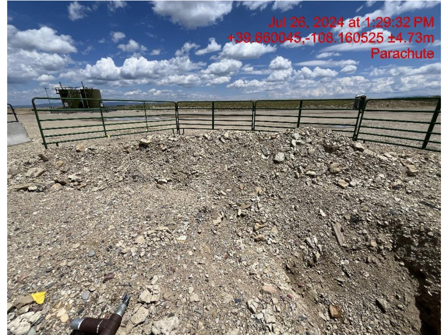
Stockpiled soils with no BMP's - Photo #03798
