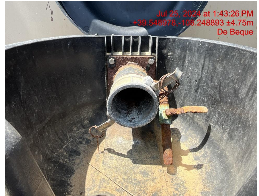
Open ended load line - Photo #03651
