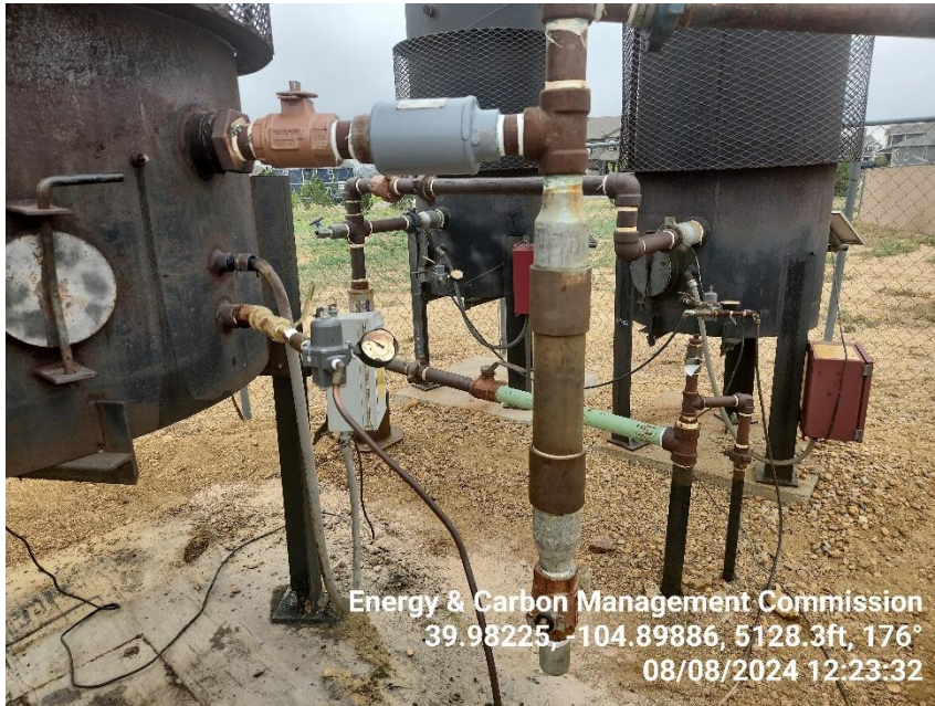
Photo 19 Damaged ECD melted wire, gauges.
