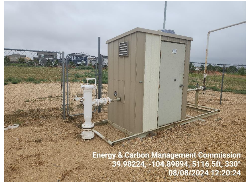
Photo 12 Gas Meter Run.
