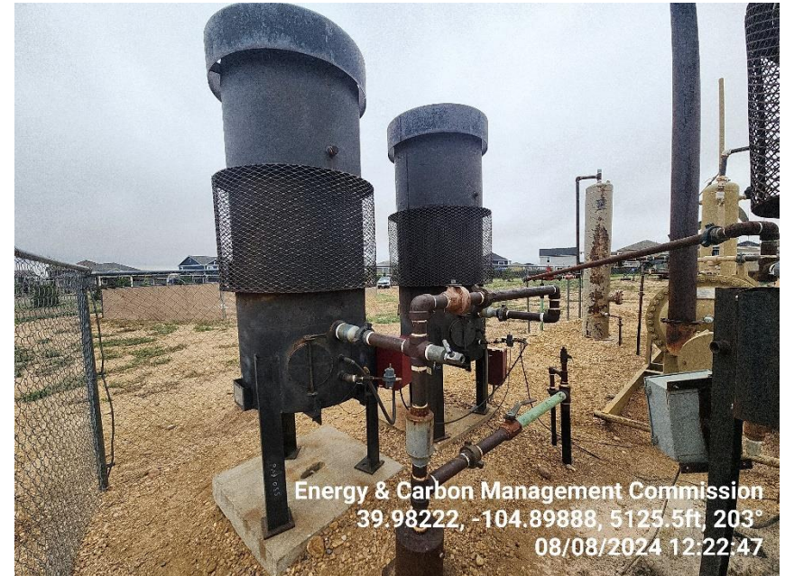
Photo 16 ECDs sight glass on pressure gages are melted.
