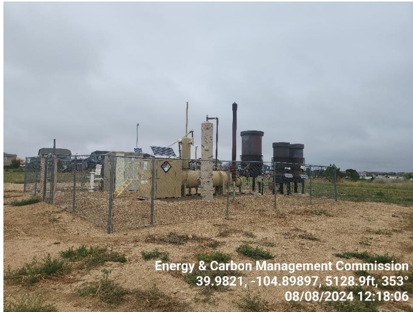
Photo 7 Gas Meter Run, ECDs & Horizontal Heated Separator.
