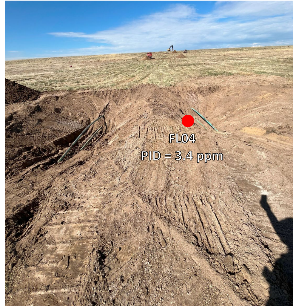
Looking west at bellhole/ cut points for removal
