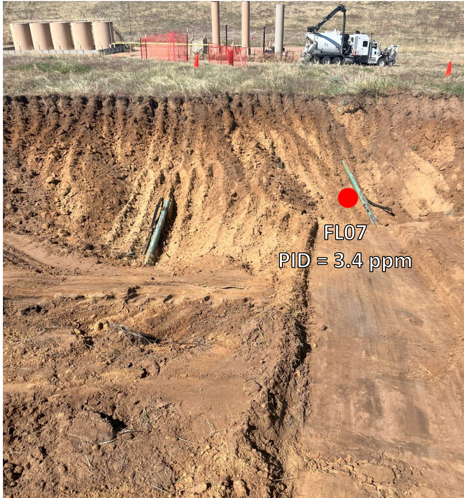
Looking west at bellholes/cut points for removal
