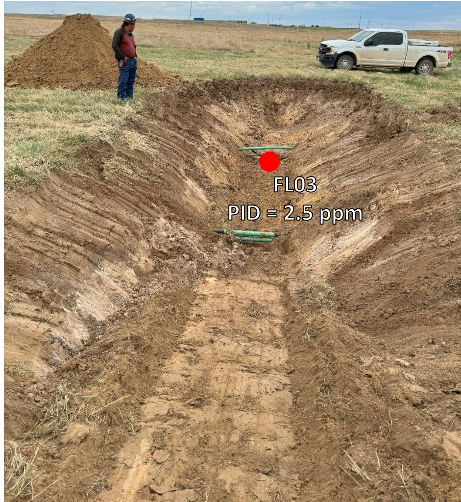
Looking north at flowline bellhole/ cut points for removal
