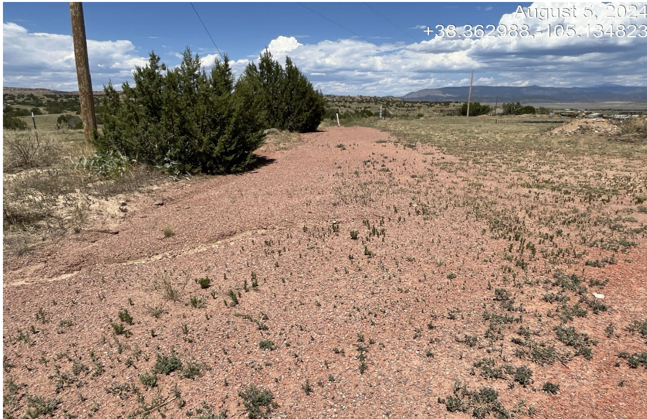
Photo 1. Facing northwest along the former access road. The red gravel was brought in by the Operator. This section of the road is now blocked by the fence and needs to be reclaimed.
