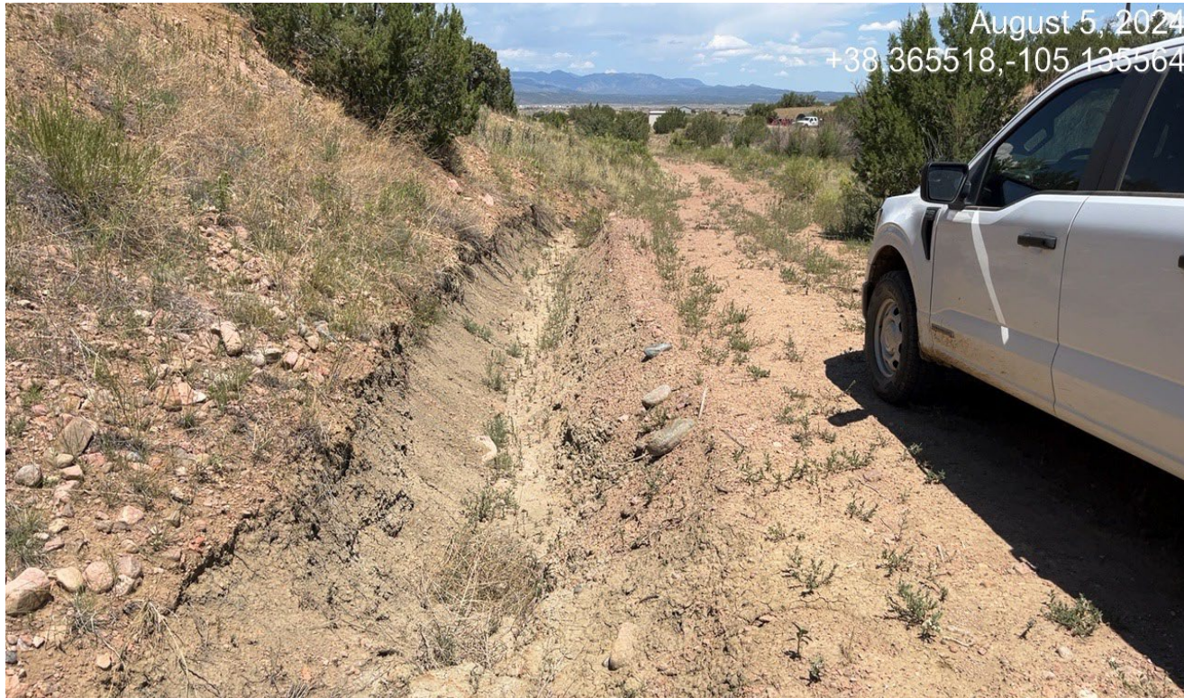
Photo 3. Facing north along the access road. There is an erosion gully along the roadside which needs to be repaired. Previous corrective action was not completed.
