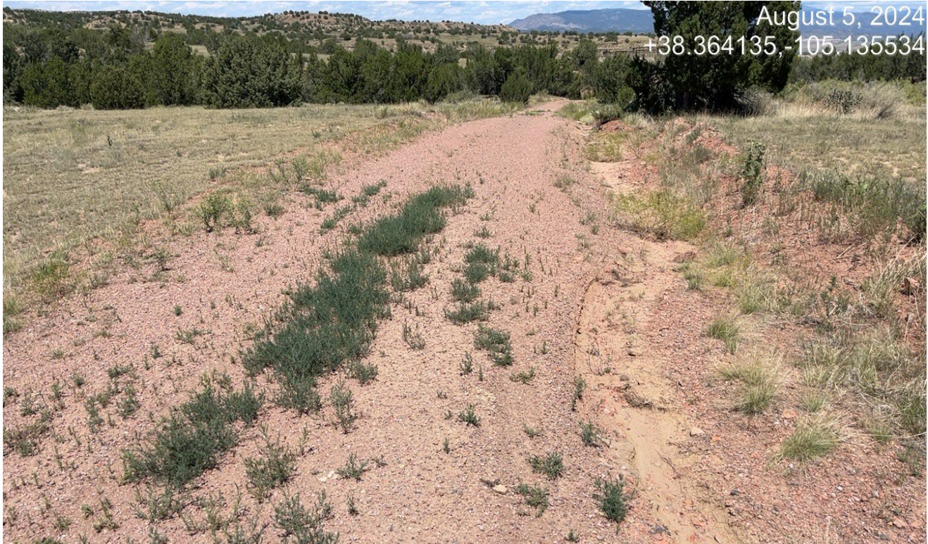
Photo 2. Facing northwest further along the access road. There is an erosion channel down the road which needs to be repaired.
