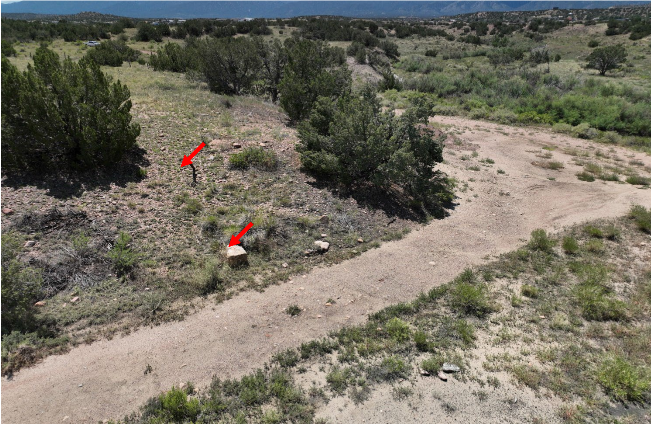
Photo 6. There is a cement block and guy line anchor that remains at the northeast side of the location which must be removed. Previous corrective action was not completed.
