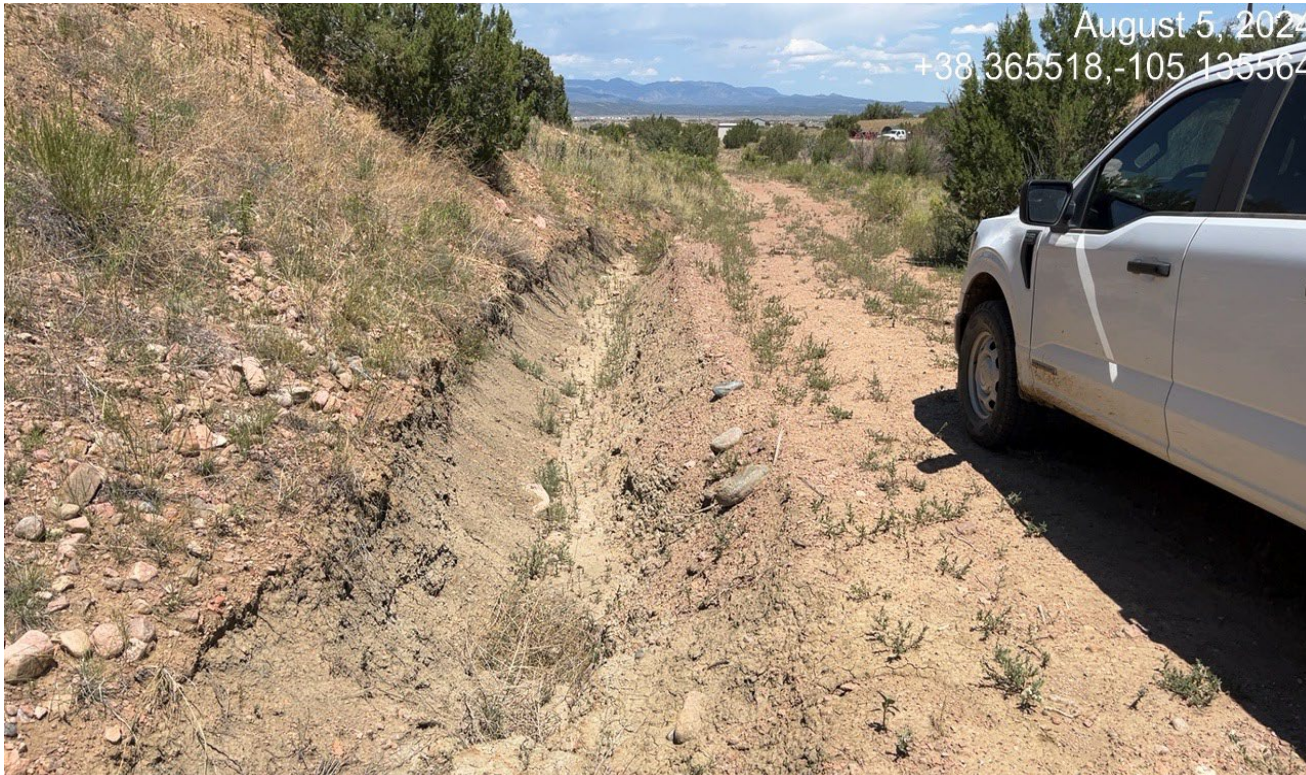
Photo 1. Facing north along the access road. There is an erosion gully along the roadside which needs to be repaired. Previous corrective action was not completed.
