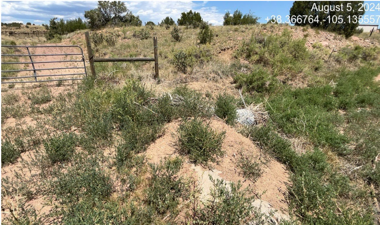
Photo 2. The culvert at this drainage crossing has filled in with sediment and debris and must be cleaned out. Previous corrective action was not completed.
