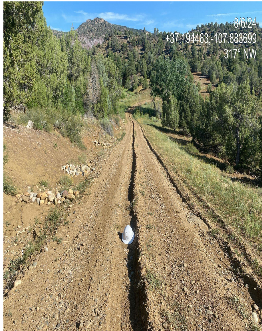
Photo 2. View of deep rutting occurring on the active pad and along the access road. Additional stabilization/grading is needed to minimize degradation to active pad/access road.
