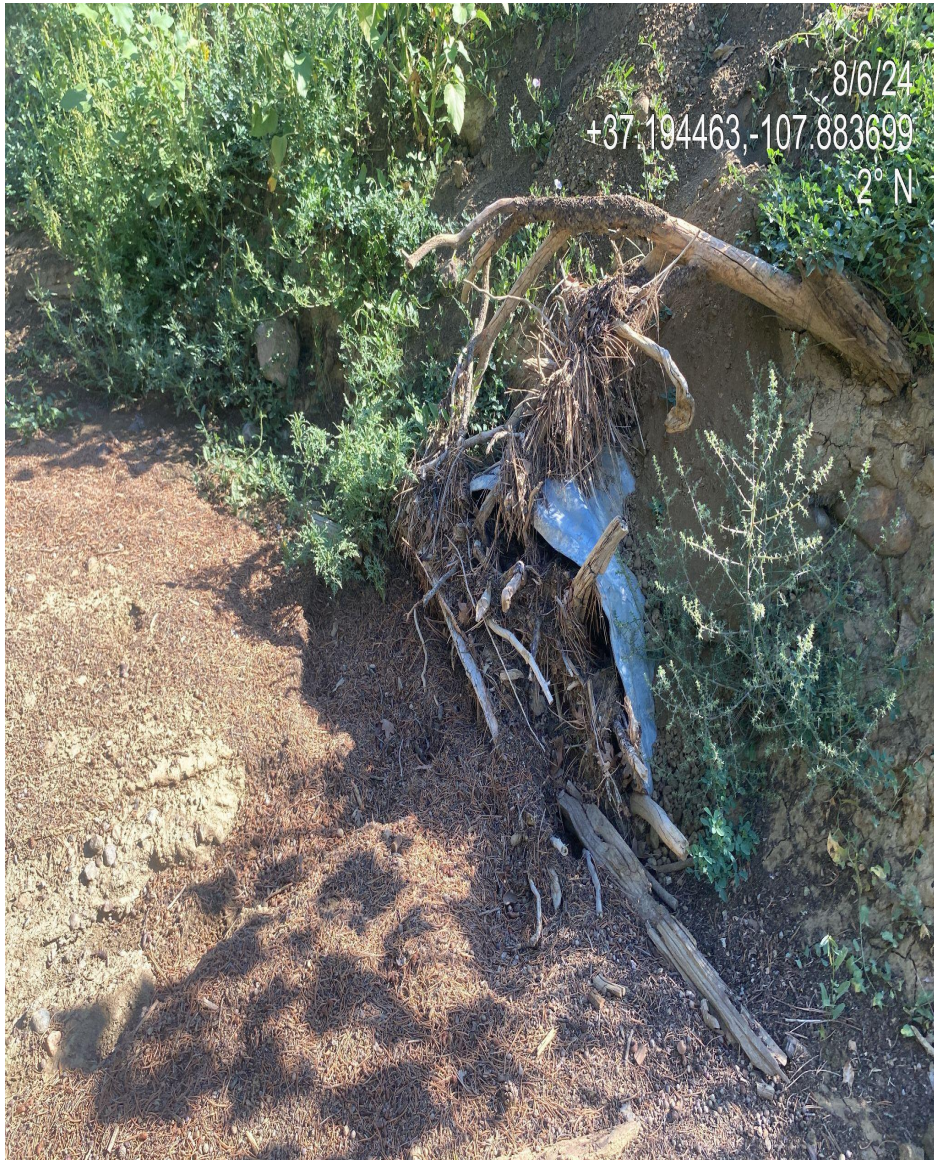
Photo 3. View of culvert crossing access road that is full of sediment/debris and is no longer functioning. Maintenance and storm water BMPs management is needed.
