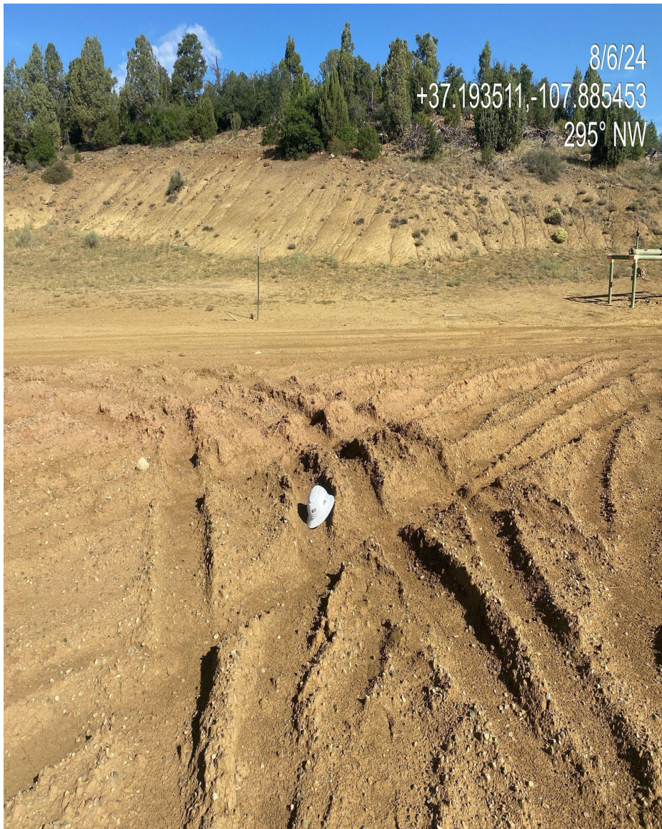
Photo 2. View of deep rutting occurring on the active pad and along the access road. Additional stabilization/grading is needed to minimize degradation to active pad/access road.
