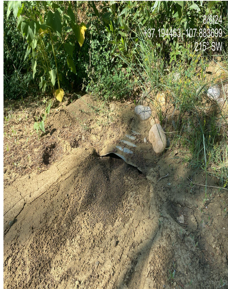
Photo 3. View of culvert crossing access road that is full of sediment/debris and is no longer functioning. Maintenance and storm water BMPs management is needed.
